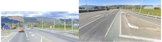
The controlled slip lane, which is set back from the Stop line on Pugh Road
