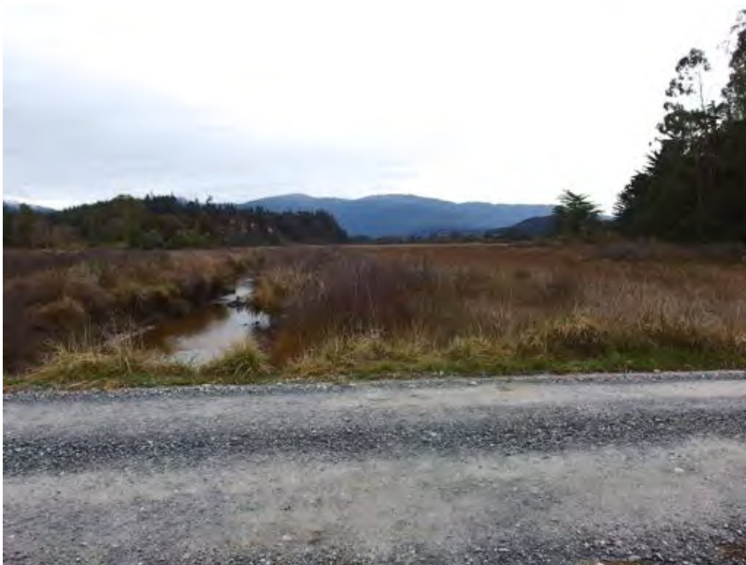
Fig. 12. View of culvert looking west to the East Arm, Motupipi Estuary
