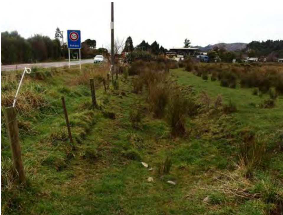
Fig. 4. View of return on bund north along Abel Tasman Drive
