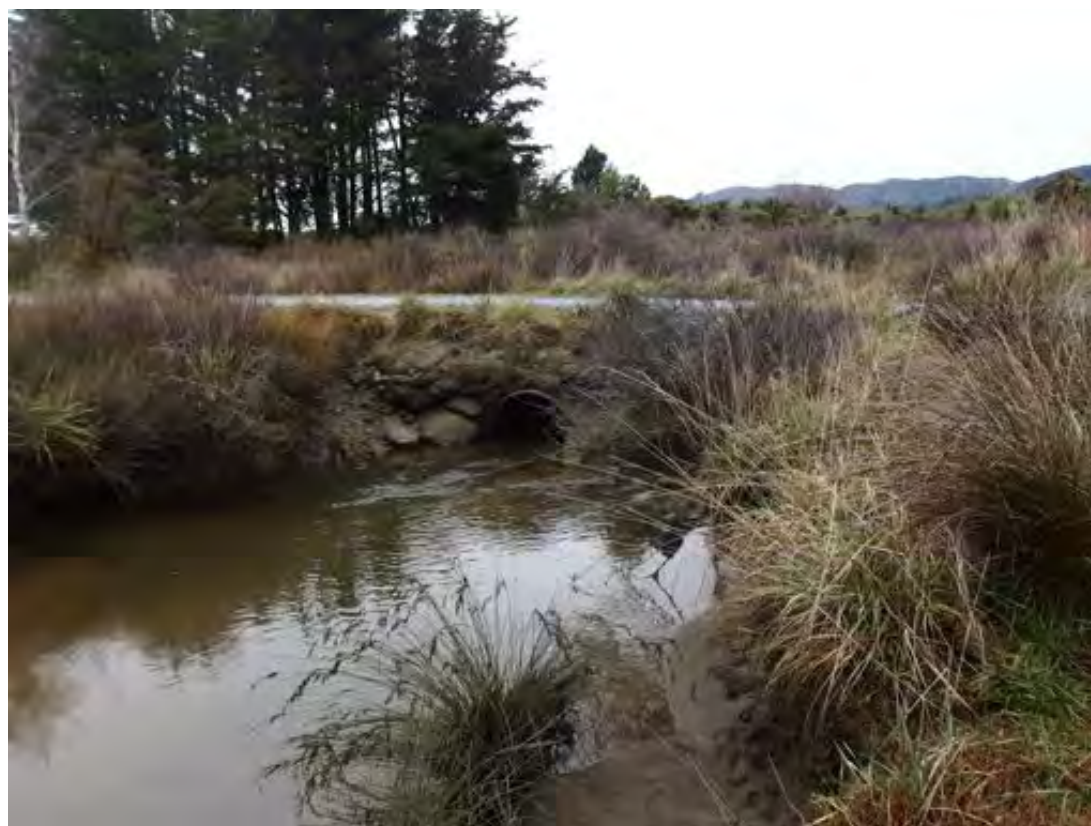
Fig. 11. View of Boyle Street culvert looking east
