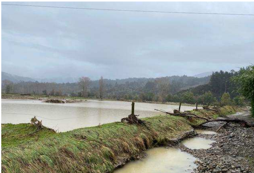
Figure 5a: Douglas Rd gravel pit scouring out neighbouring boundary during flood. Photo taken the day after 17.7.21 flood.
