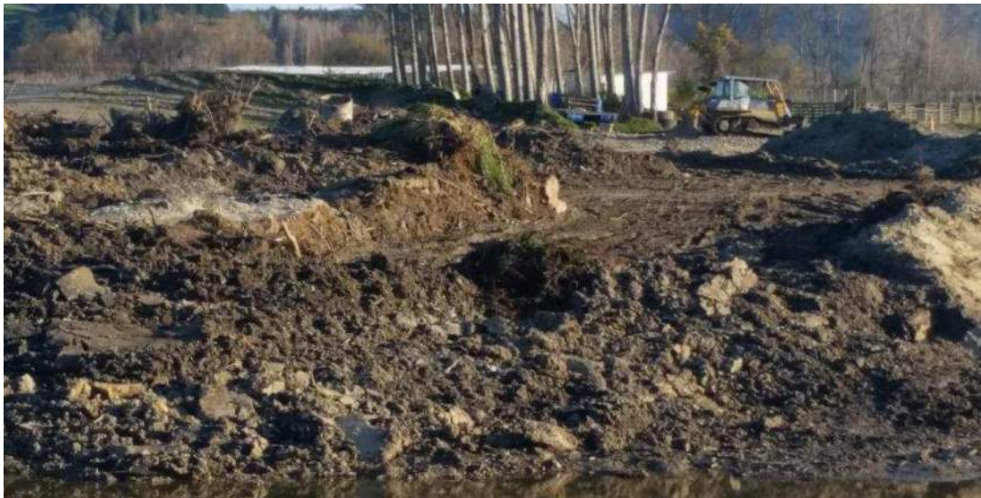
Figure 1: A typical industrial scale gravel extraction operation- Douglas road.
