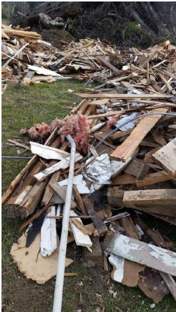
Figure 2: Demolished house and parts dumped for disposal- Douglas Road. Photo taken 18.7.20
