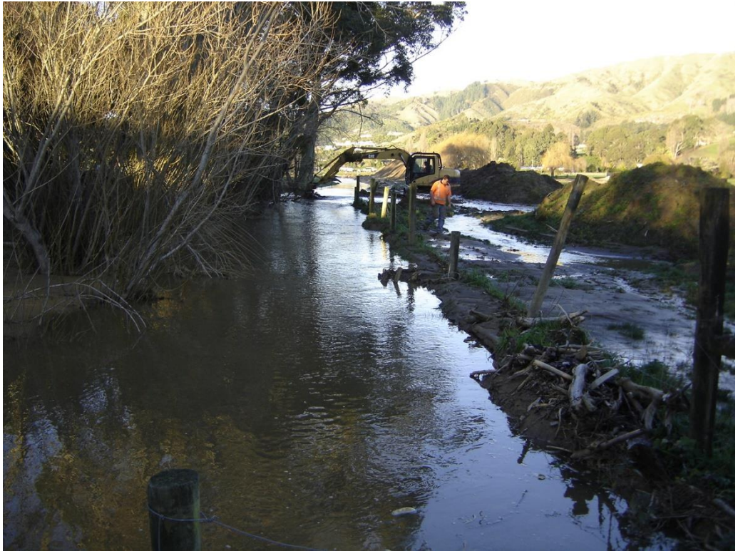
Photo 5: Ellis Creek channel clearance upstream of 59a Selwyn Street, July 2012
