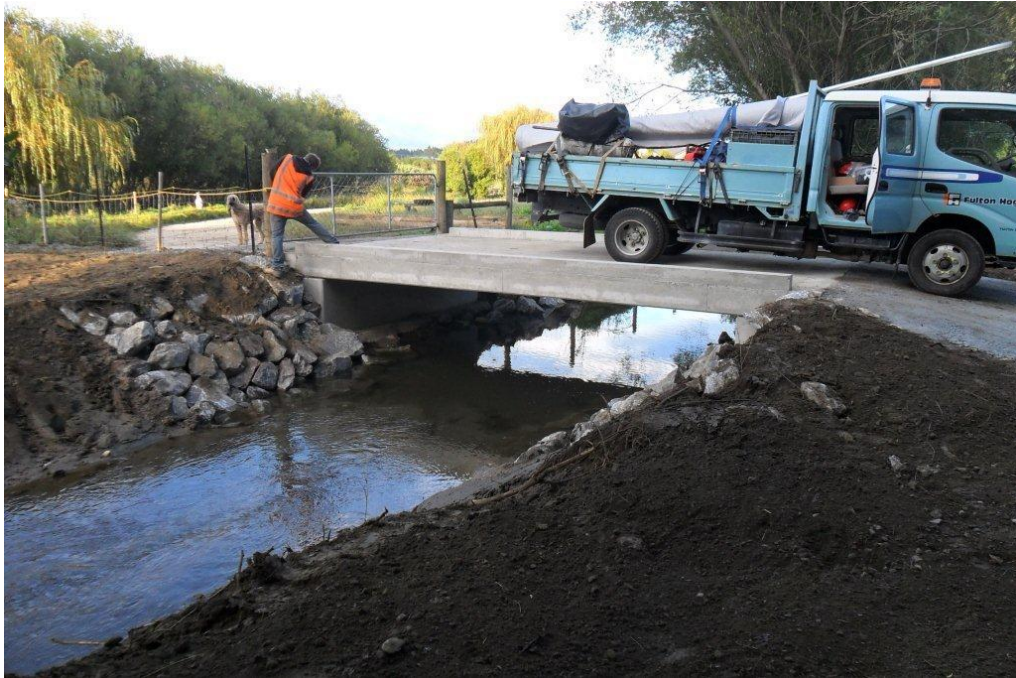
Photo 8: New bridge on Ellis Creek at 59a Selwyn Street, March 2013
