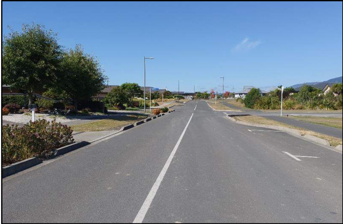
Figure 3: Fairrose Drive with no landscaping.
