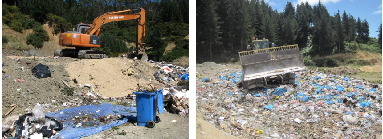
Figure 4-4: Excavator and compactor used at York Valley Landfill
