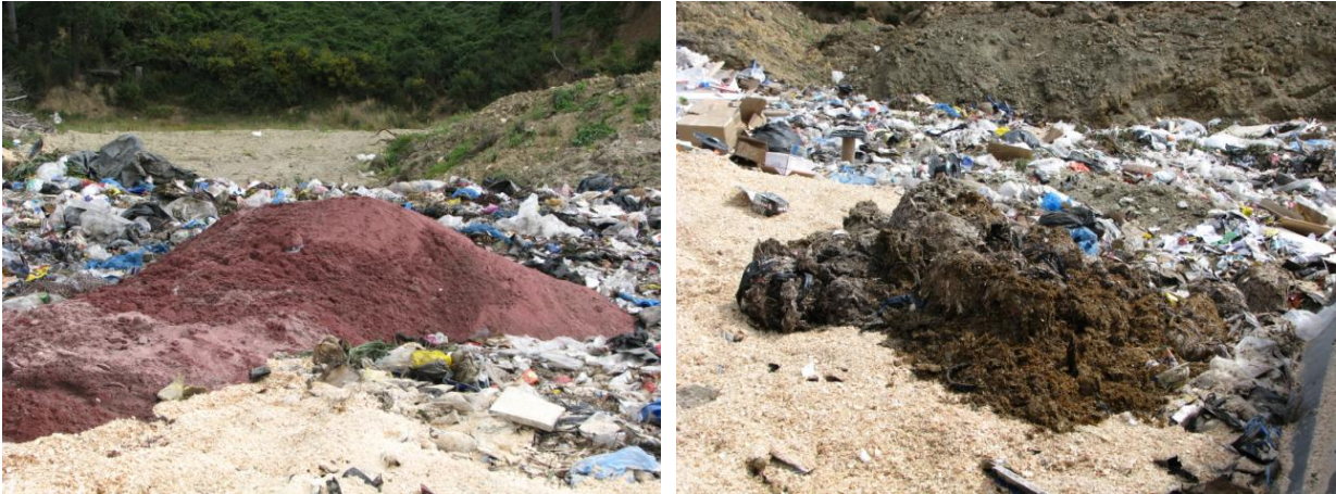
Figure 5-2: Examples of uniform loads observed at York Valley Landfill
