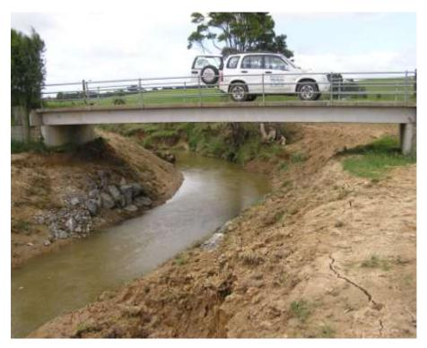
Figure 14 Typical single span farm bridge
