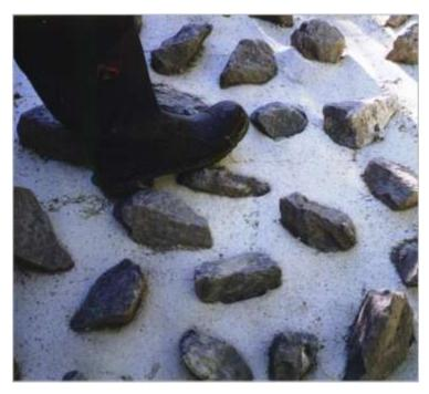
Figure 10 Rocks can be cemented into the base of waterway crossings and/or to the aprons of culverts to ensure that there are areas of low water velocity available to aid fish passage and sediment which is appropriates for invertebrates is retained within the structure
