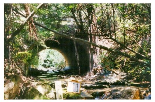
Figure 2 Single barrel arch culvert
