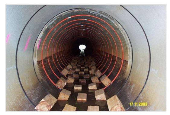
Figure 9 Baffles (these can be of many materials) and rocks can be installed into the base of a waterway crossing to provide cover and low velocity zones to aid with fish passage
