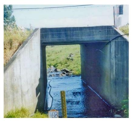
Figure 8 Single box culvert
