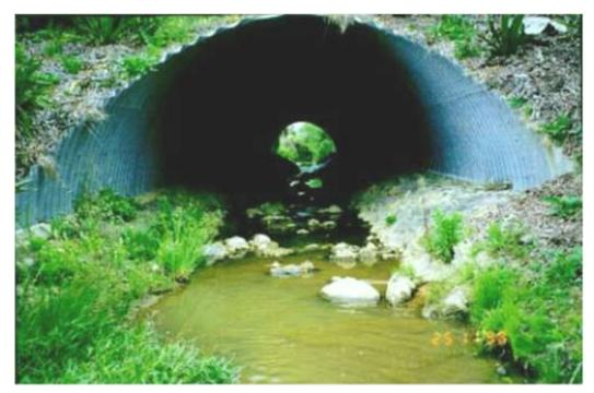
Figure 3 Best Practice - single barrel arch culvert
