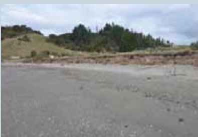
Low eroding terrace at Onahau
