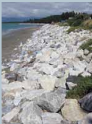
Coastal erosion protection, Ruby Bay
