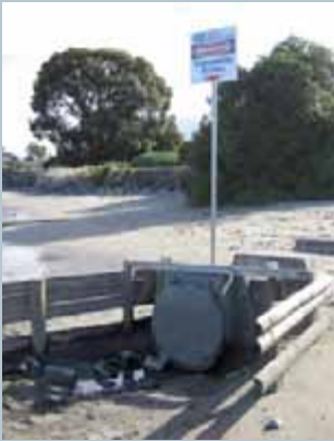
Stormwater outfall, Moutere delta
