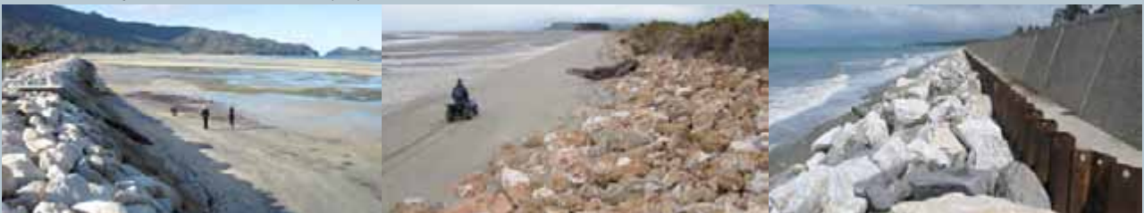
Seawalls - left to right at Marahau, Waikato, and Ruby Bay
