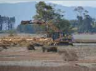
Road causeway being removed - Moutere Inlet, 2010
