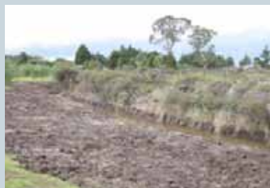
Drainage of the northern terrestrial margin.
