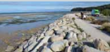
Seawall at Marahau Beach
