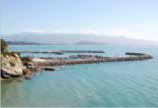
Tarakohe Harbour breakwater
