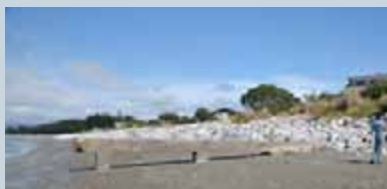
Rockwalls and stormwater outfall, Ruby Bay Beach.
