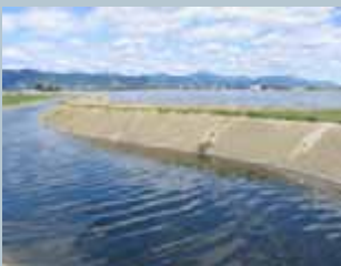
Bells Island wastewater ponds, Waimea Inlet
