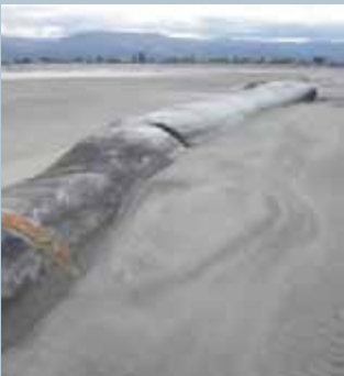
Geotextile groyne - Moutere Delta
