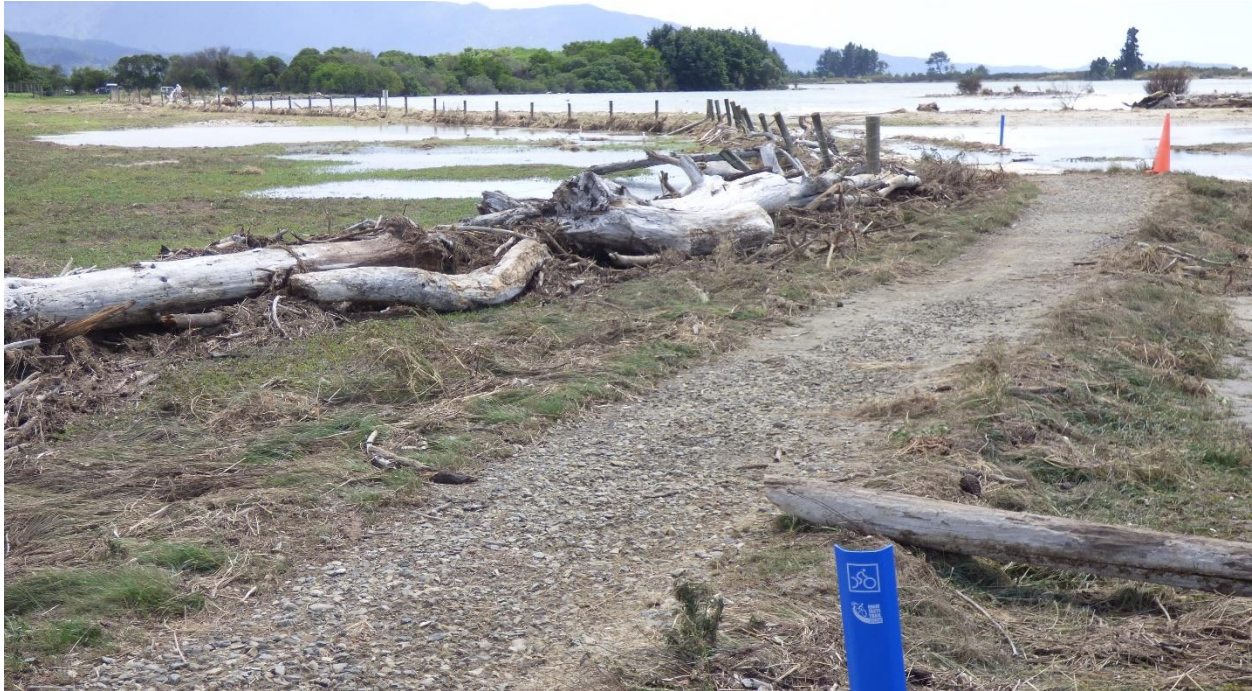
Figure 40. Storm surge damage and inundation, Tasman Bay, February 2018. [D.S. Melville]
