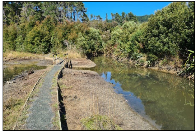
Constructed channel west of the embayment, which first appeared in aerials in the 1980s. The Kimi Ora Resort pathway follows the embayment's western margin.
