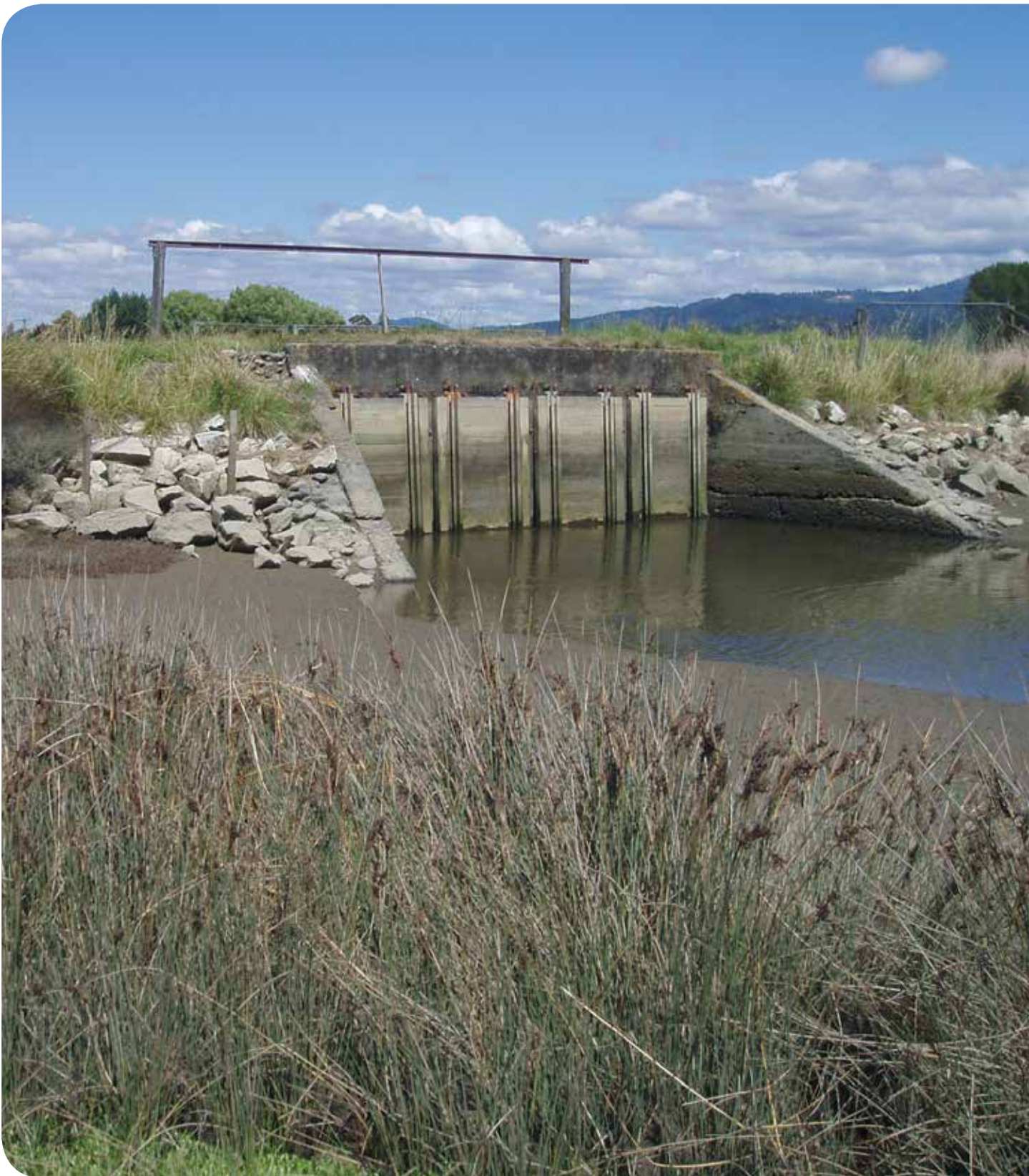
Tidal gates prevent the passage of whitebait and interfere with spawning.
