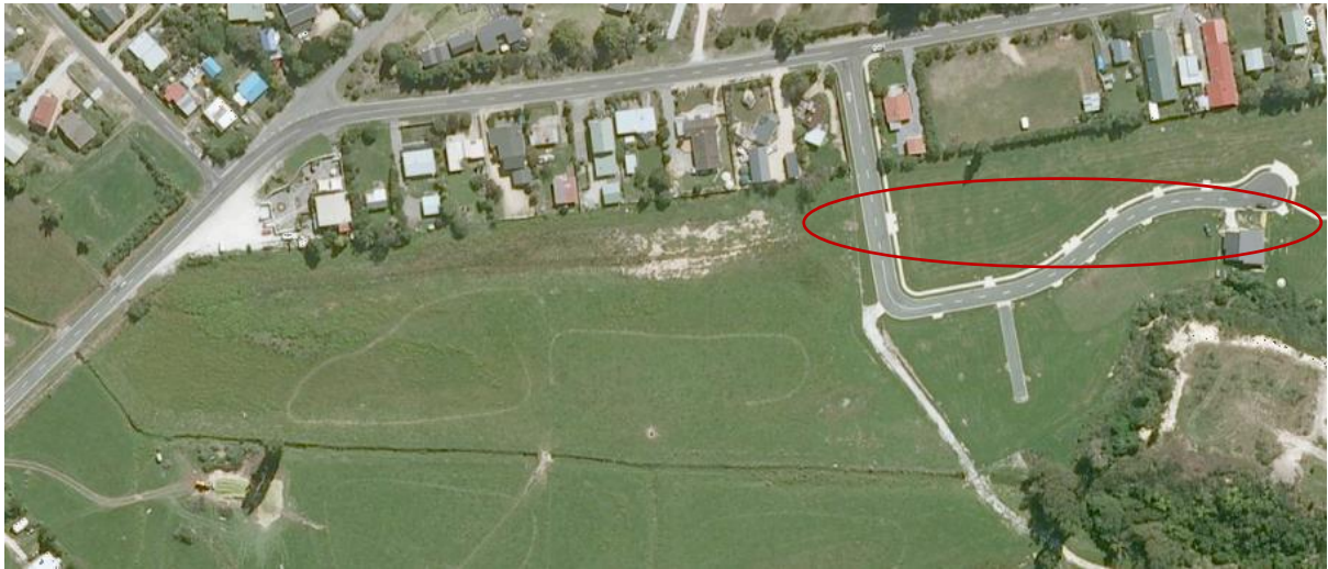
Figure 3: Aerial image – 2007 (Council GIS). Shows the blocking of the drain. As built plans suggest the outlet was raised to an RL of 3.15 m
