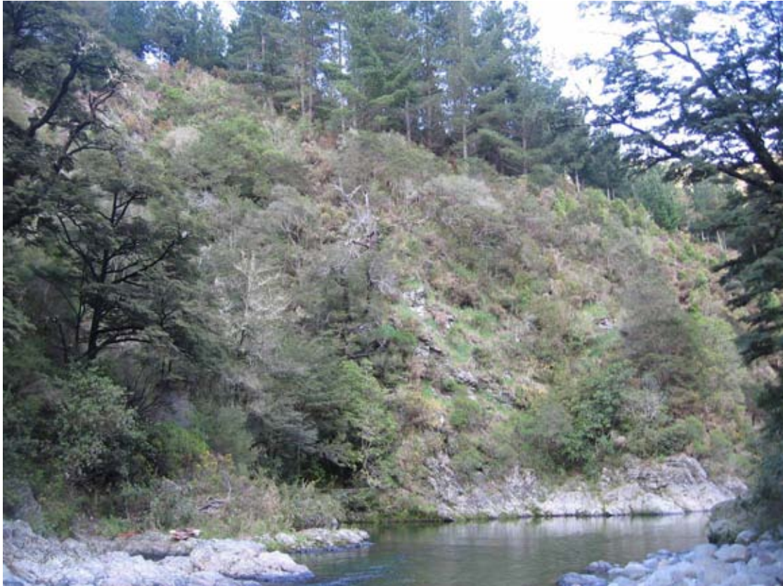
Photo 8: Downstream of centreline, left abutment foundation
