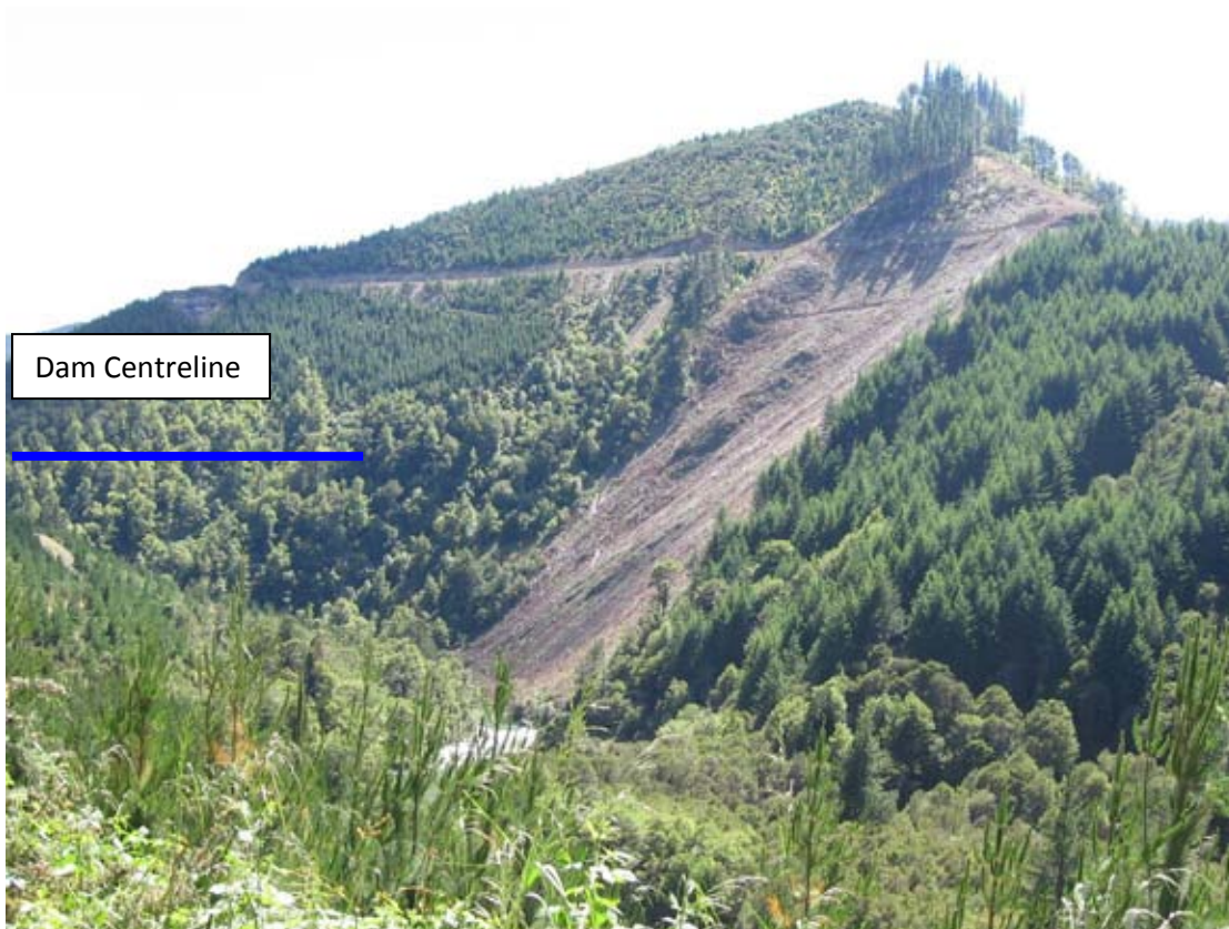
Photo 3: View of left abutment slope
