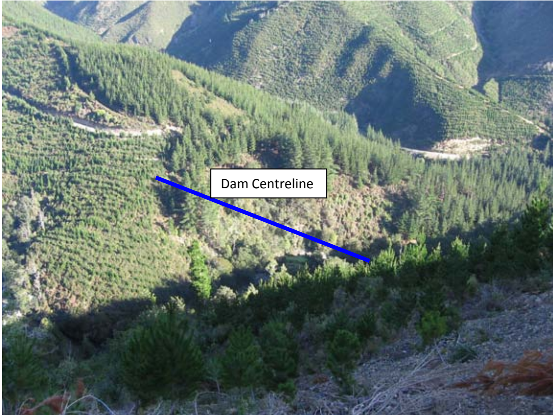
Photo 2: Dam Left abutment
