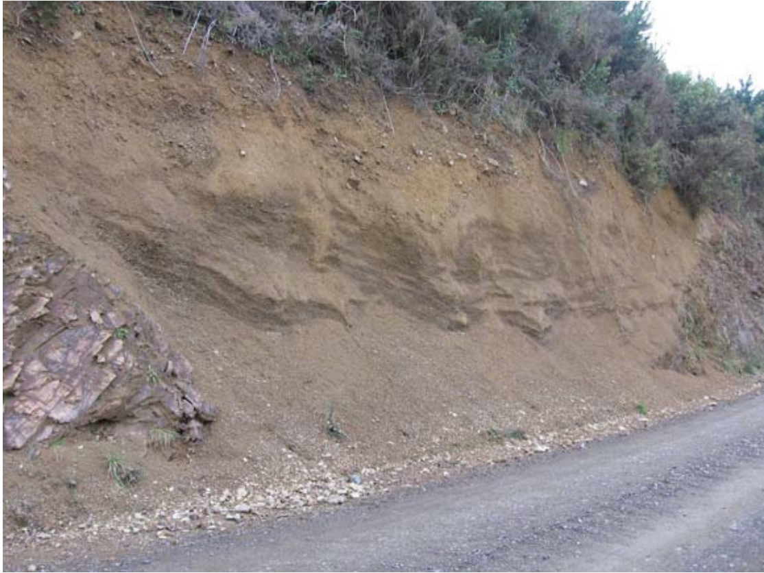
Photo 12: Solifluction deposit infilling fossil gully, upstream of left abutment
