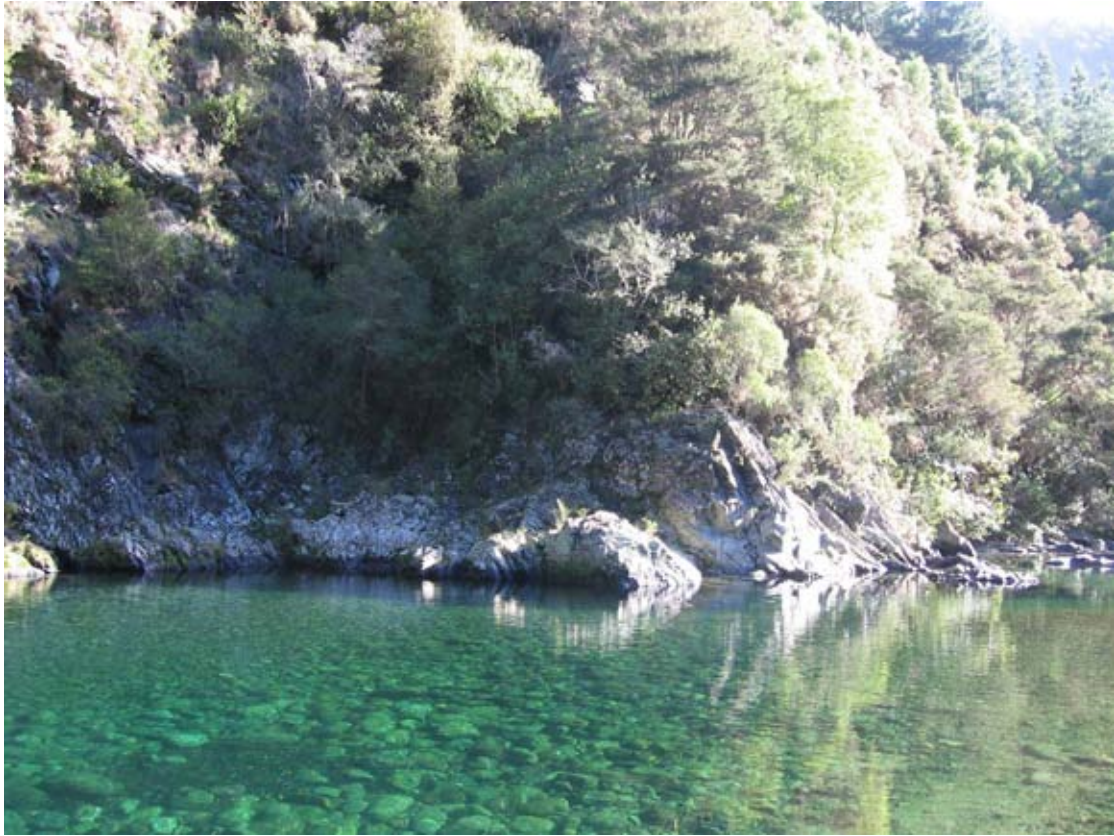
Photo 8a: Downstream left abutment near dam toe (closer view of Photo 8)
