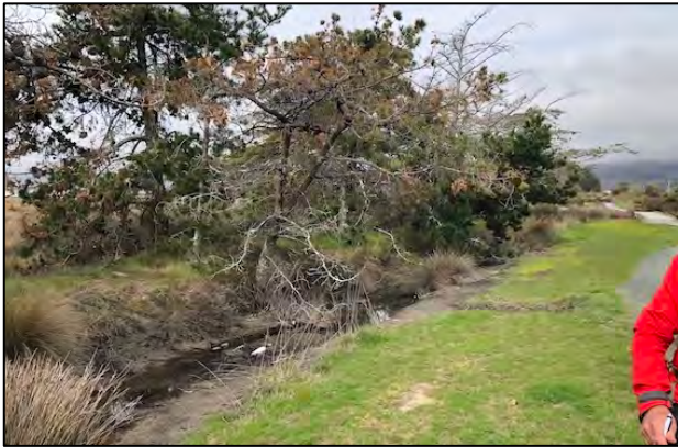
Pine trees growing on an earth bund seaward of a drainage channel running parallel to the shore
