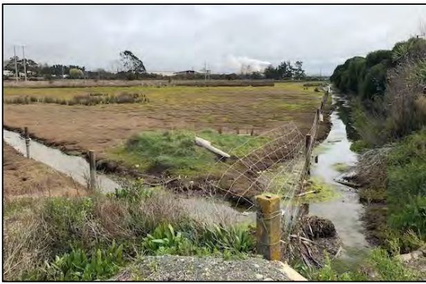
Grazed salt marsh cut off from the sea by a large earth bund (right) and channelising to drain water
