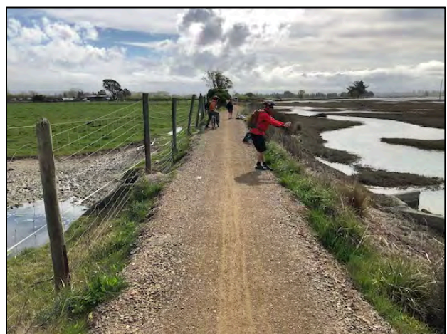
Farmland at the same tidal elevation as the estuary, but separated by an earth bund that restricts tidal inundation
