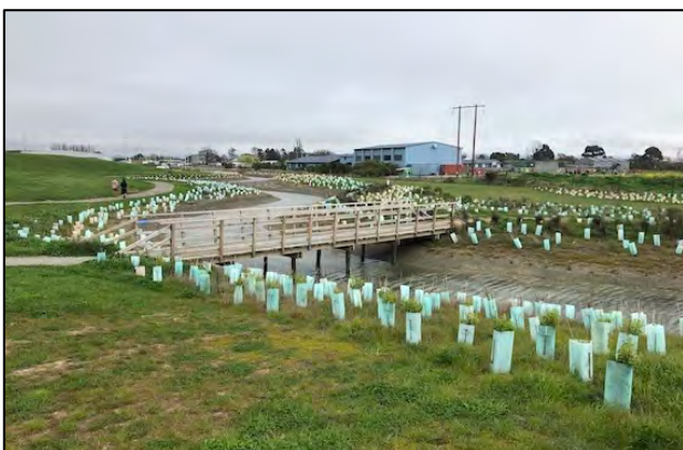
Meanders were built into the lower streamway and the edges reshaped to have a gentle slope prior to planting
