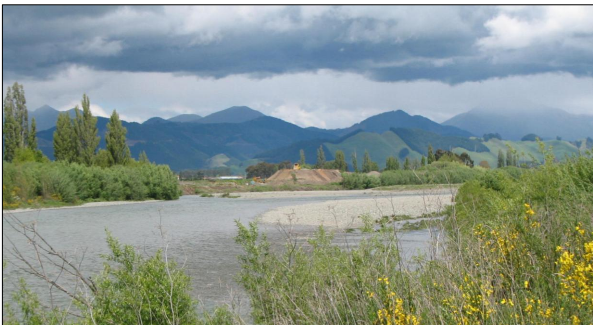
Stock pile at gravel-processing plant
