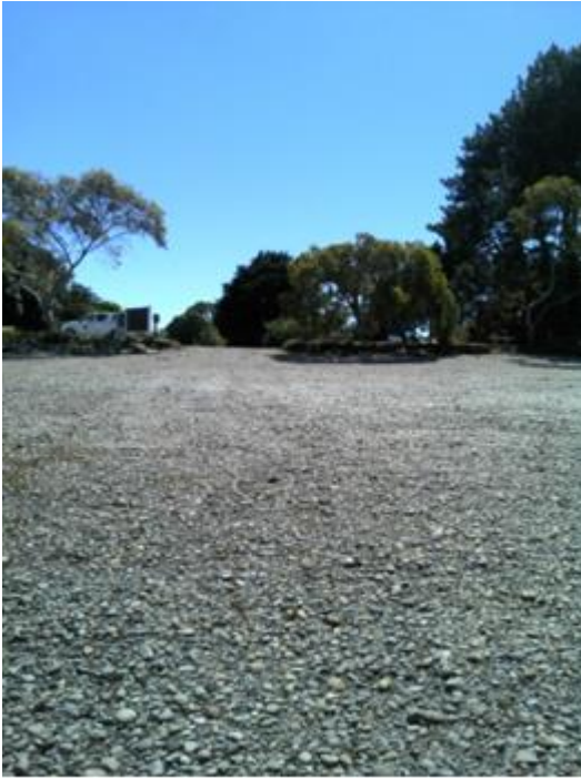
Figure 12: Grossi Point Boat Ramp
