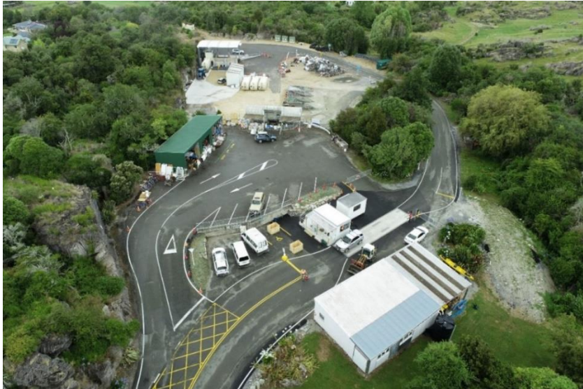
Figure 17: Tākaka RRC – recycling drop-off and reuse shop in foreground, with waste compactor, scrap metal and greenwaste drop-off in background
