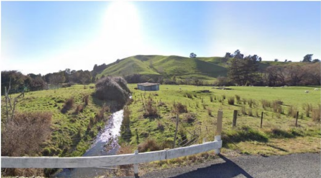
Photograph 2 – Gossey Creek looking downstream from the bridge across Edward Street (Source: Google Street View)
