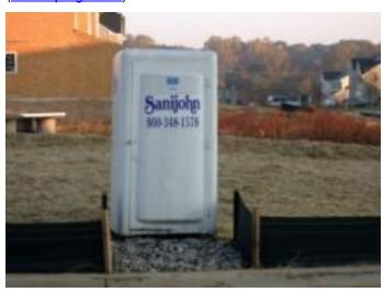
Figure 10-2 Good example of a port-a-loo placed in a location with consideration also given to erosion and sediment controls
