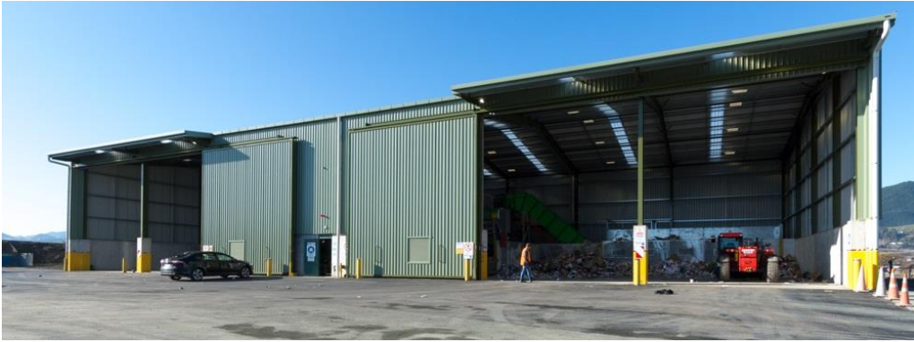
Figure 2: Exterior Photo of Richmond RRC
