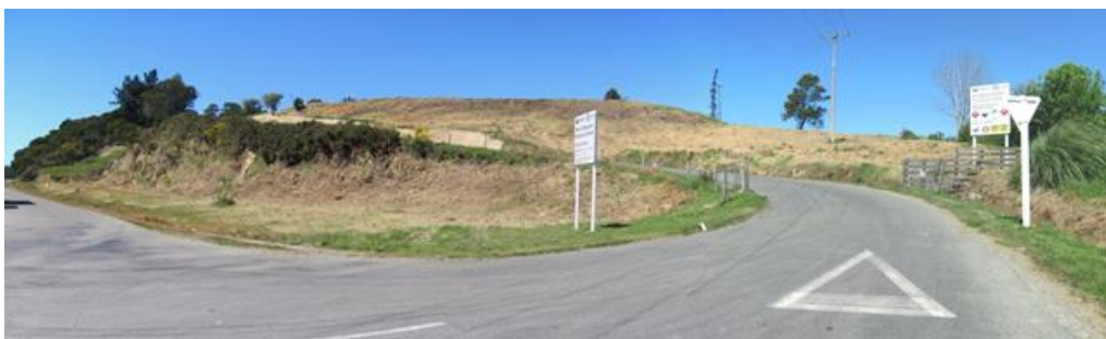
Figure 6: Mariri RRC – Entrance from Robinson Road
