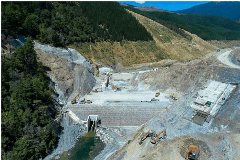
Figure 3: Downstream overview of layer-12 of the reinforced rockfill being placed, 3 Feb 2021
