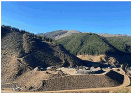
Figure 32: Stock pile of blended 2B material
