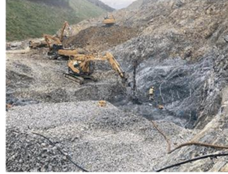
Figure 31: Removal of unsuitable material
