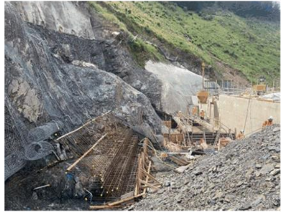
Figure 14: RHS plinth void buttress support concrete pour, Nov 2020
