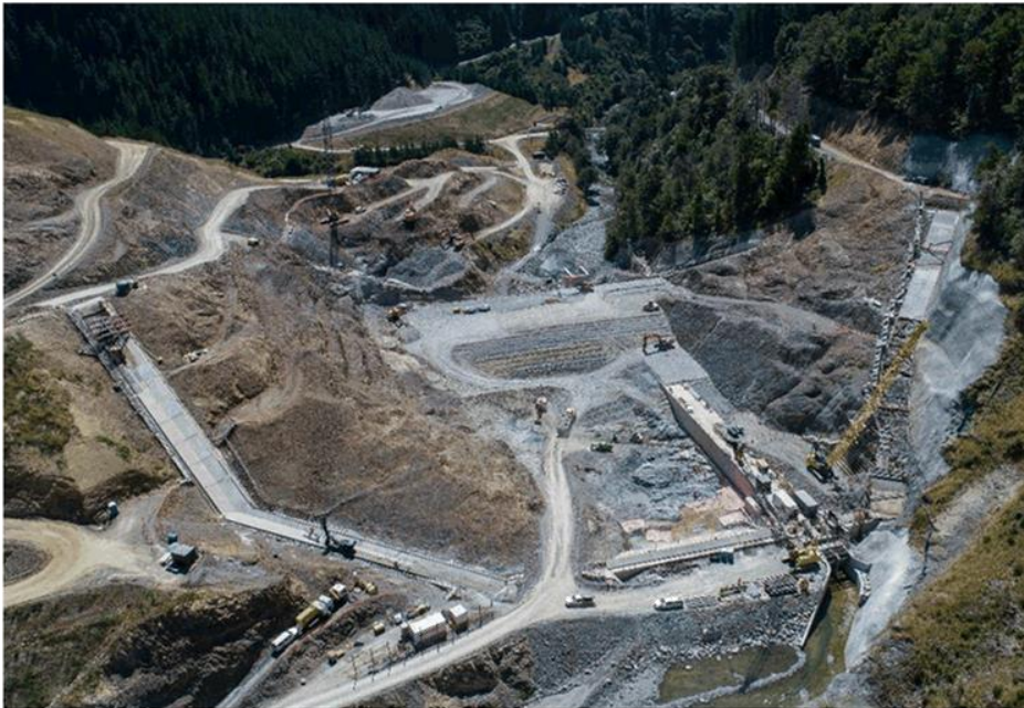
Figure 17: Overview of the dam footprint, looking downstream, Feb 2021
