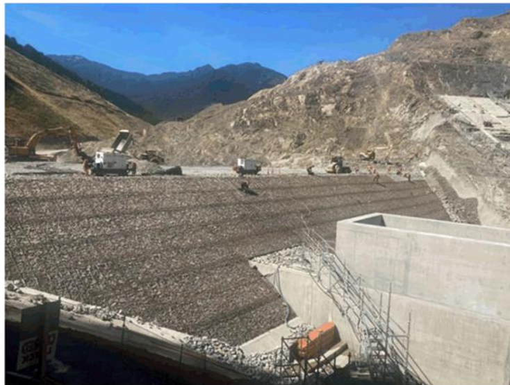
Figure 10: Reinforced rockfill, 2 February 2021
