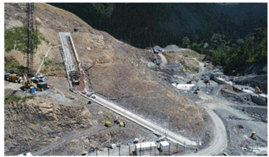
Figure 16: LHS plinth progress looking downstream, Dec 2020
