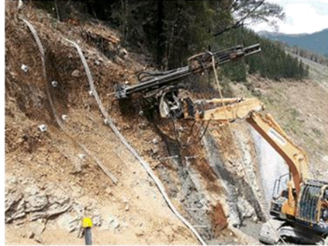
Figure 34: Colluvium stabilisation
