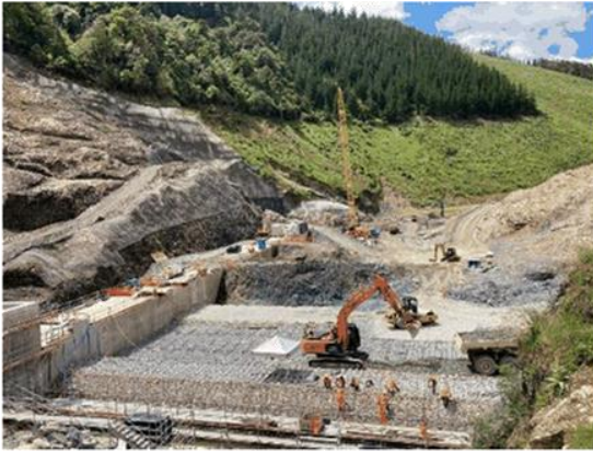
Figure 11: Overview of reinforced rockfill placement, Dec 2020
