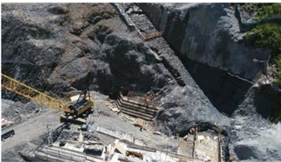
Figure 15: Overview of RHS plinth foundation and void, Dec 2020
