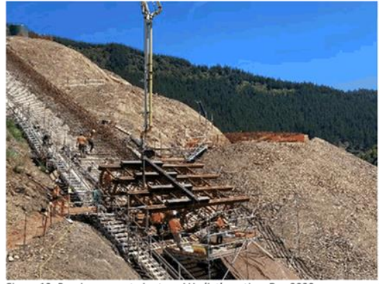
Figure 12: Pouring concrete in steep LH plinth section, Dec 2020
