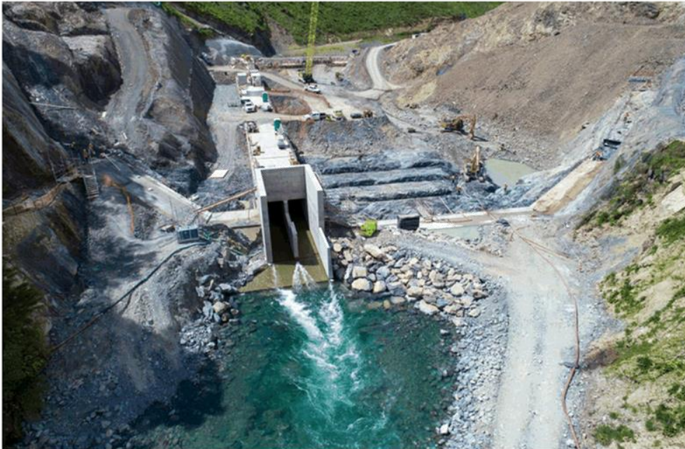
Figure 18: Clean water flowing through the diversion culvert as site works continue
