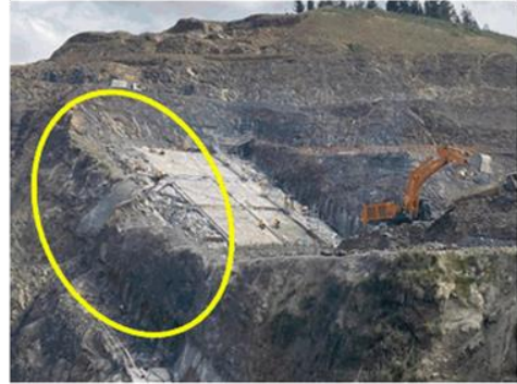
Figure 35: Stabilisation beneath the spillway
