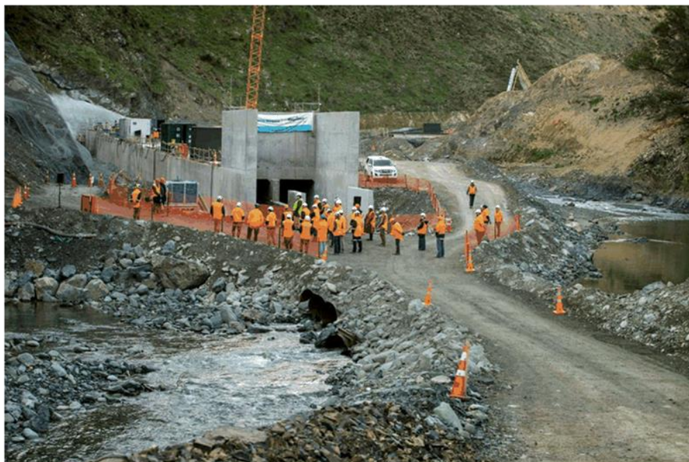
Figure 1: Diversion Culvert Blessing, August 2020
