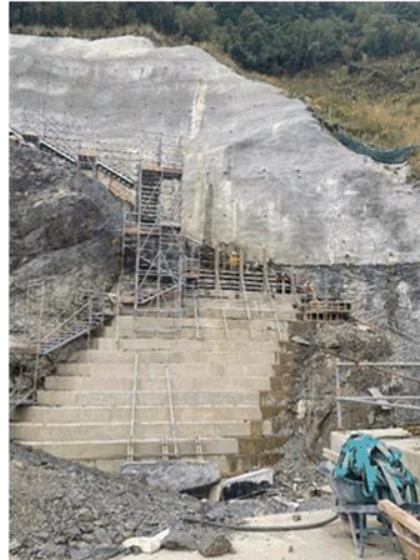
Figure 40: Buttress wall and beam
