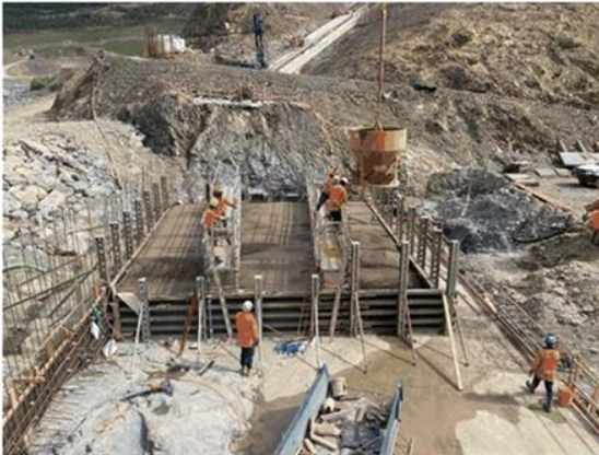
Figure 13: Pouring concrete in starter dam, Nov 2020
