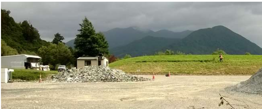
Figure 9: Murchison RRC – Recycling Shed on Left Background and Closed Landfill to the Right
