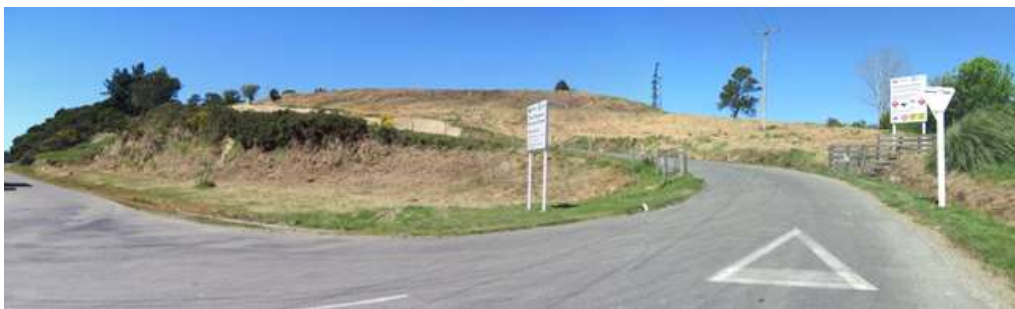
Figure 6: Mariri RRC – Entrance from Robinson Road
