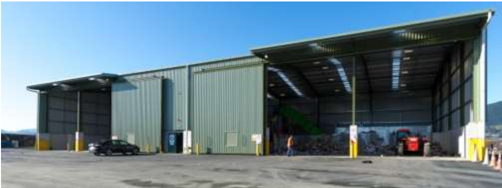
Figure 2: Exterior Photo of Richmond RRC
