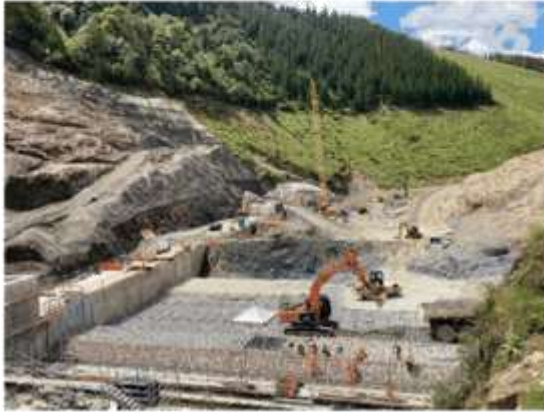
Overview of reinforced rockfill placement, Dec 2020
