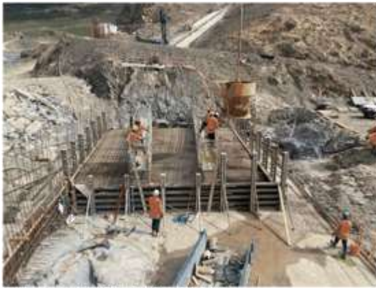
Pouring concrete in starter dam, Nov 2020
