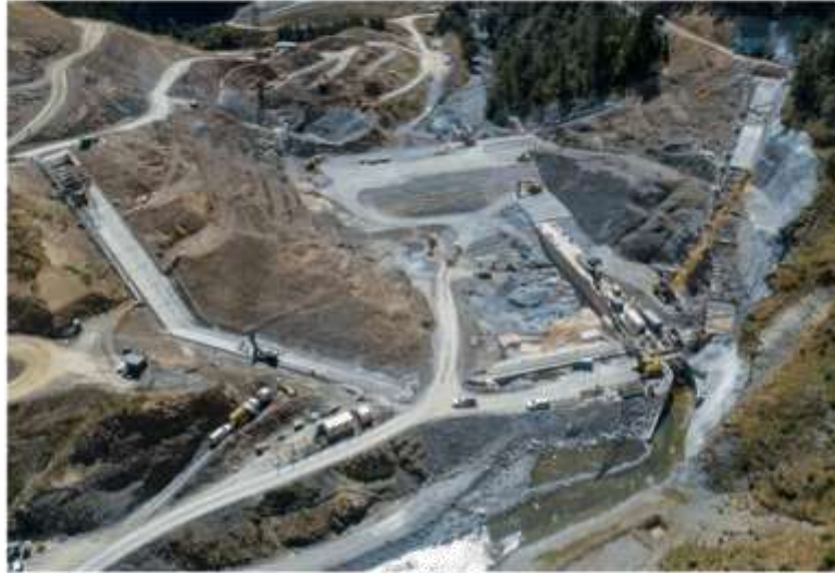
Aerial view of the site progress, February 2021
