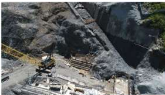
Overview of RHS plinth foundation and void, Dec 2020
