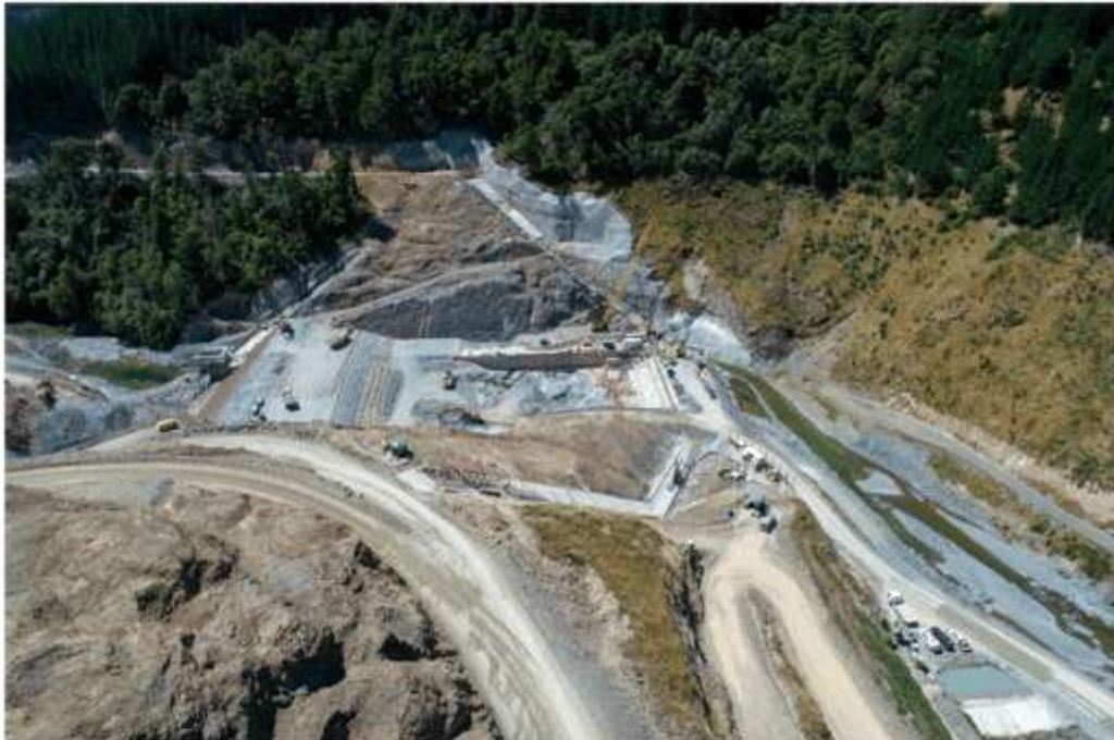
Construction Site, February 2021
