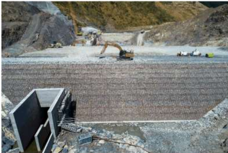
Downstream view of rockfill embankment
