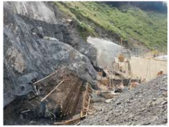
RHS plinth void buttress support concrete pour, Nov 2020
