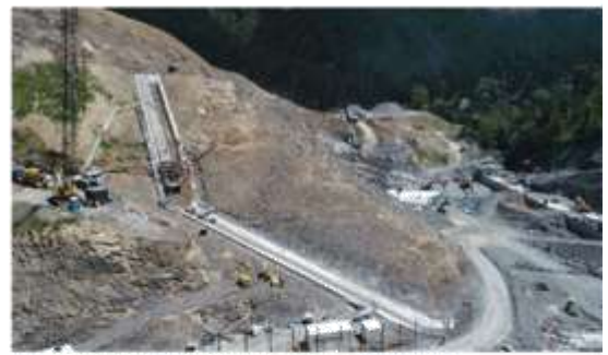
LHS plinth progress looking downstream, Dec 2020
