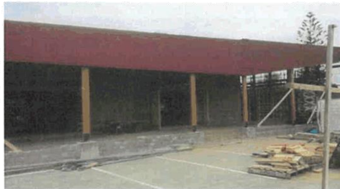
Roof facade completed, 20 April
