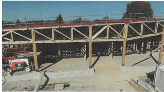
View from the carpark showing the main entrance, 22 March
