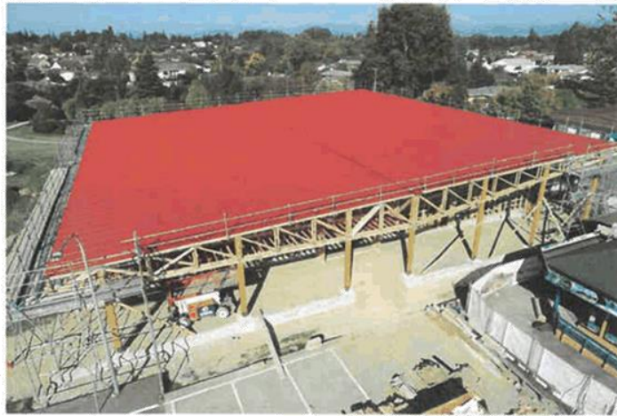
Roof close to completion, 22 March
