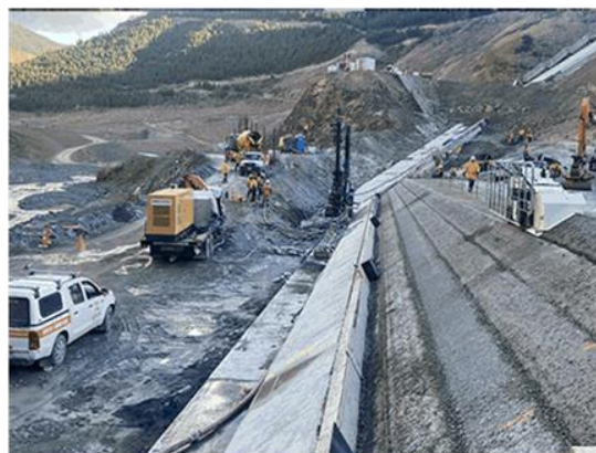
Figure 14: LH abutment foundation treatment & kerb placement
