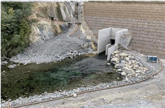
Figure 17: Clean, clear water flowing from the diversion culvert
