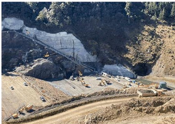
Figure 9: Overview of the embankment footprint from top of Spillway
