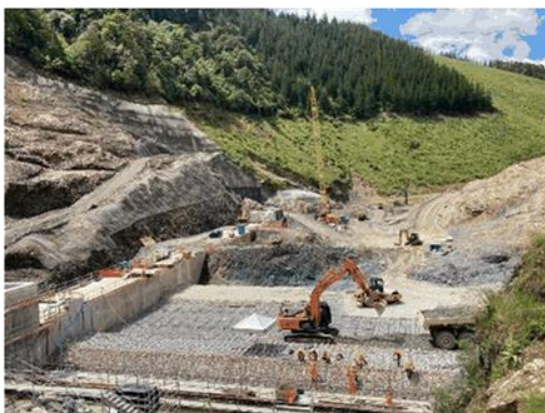
Overview of reinforced rockfill placement, Dec 2020
