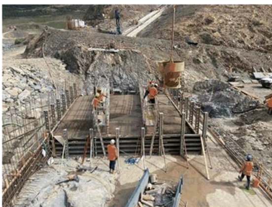
Pouring concrete in starter dam, Nov 2020
