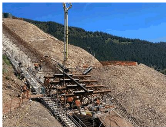
Pouring concrete in steep LH plinth section, Dec 2020
