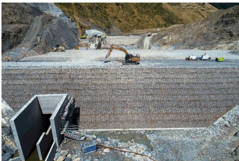
Downstream view of rockfill embankment
