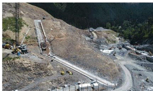
LHS plinth progress looking downstream, Dec 2020
