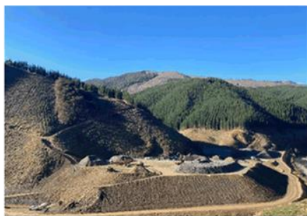
Stock pile of blended 2B material
