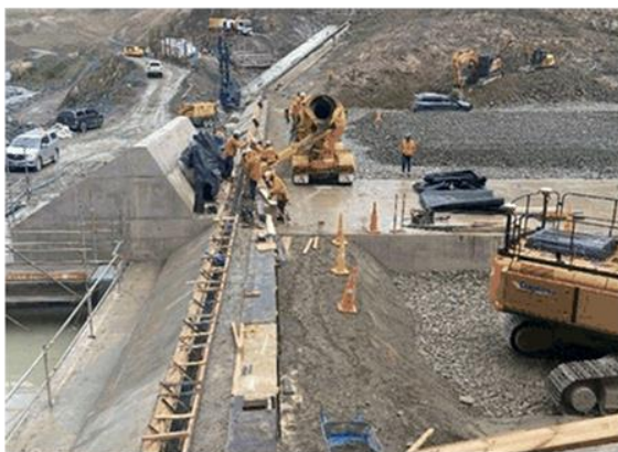
Figure 13: The first hand-made kerb is being placed
