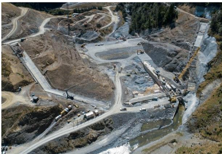
Aerial view of the site progress, February 2021
