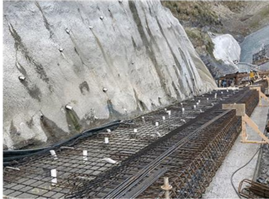
Figure 16: Steel fixing progress on RH plinth
