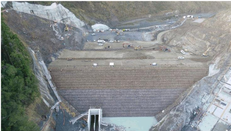
Figure 1: Reinforced Rockfill embankment viewed from downstream. Culvert on the left-hand side and spillway on the right of photo.
