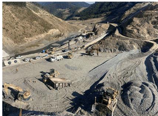
Figure 10: Upstream third embankment filling progress
