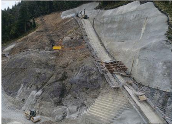
Figure 15: RH plinth concrete complete. Drilling anchor holes at top
