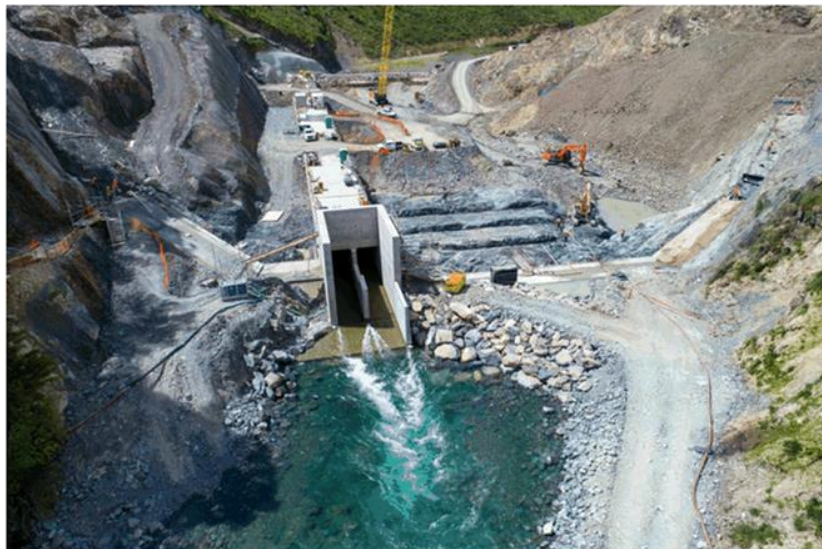
Clean water flowing through the diversion culvert during construction works
