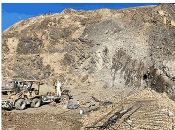
Figure 11: Preparing the last section of LHS downstream anchor slab
