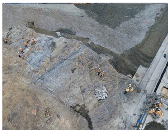
Figure 12: Cleaning LH abutment foundation
