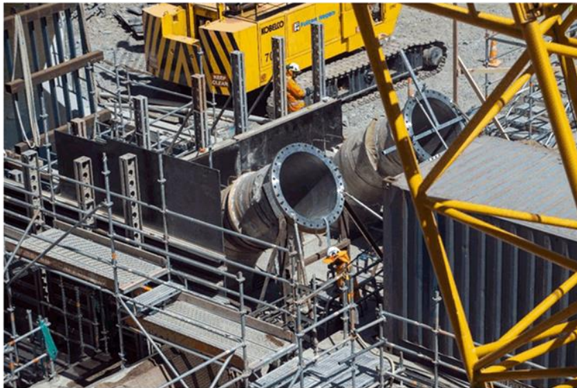
The first part of the dam's outlet works
