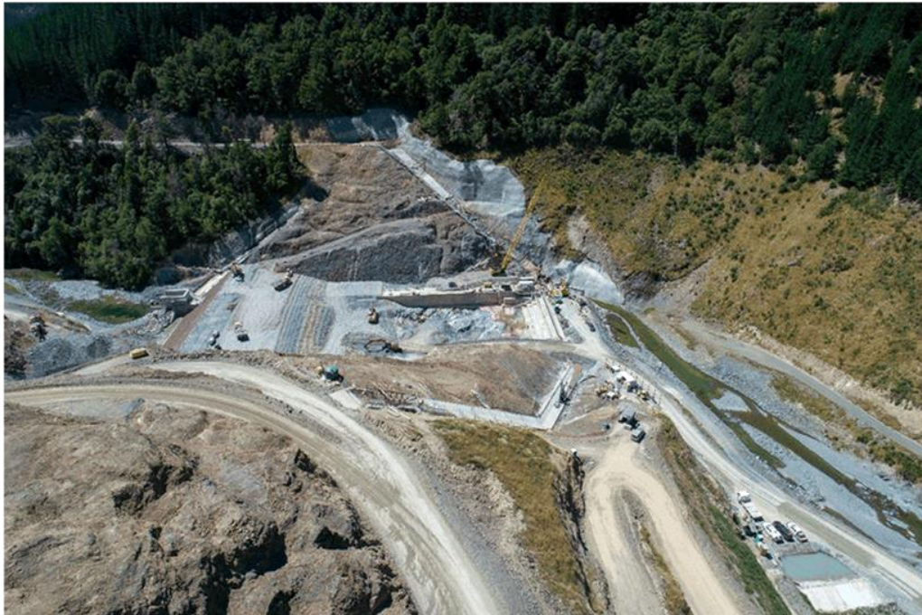
Construction Site, February 2021
