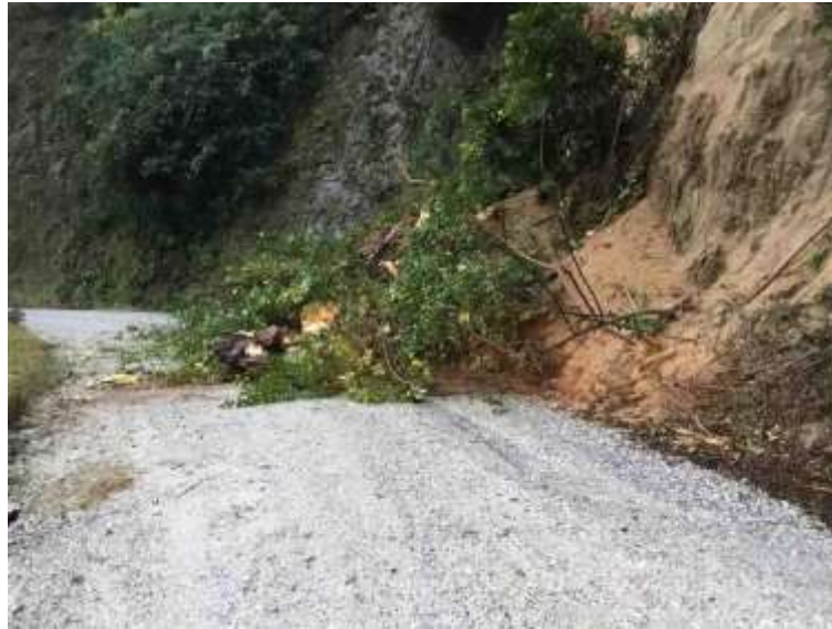
Tataranui Road slip
