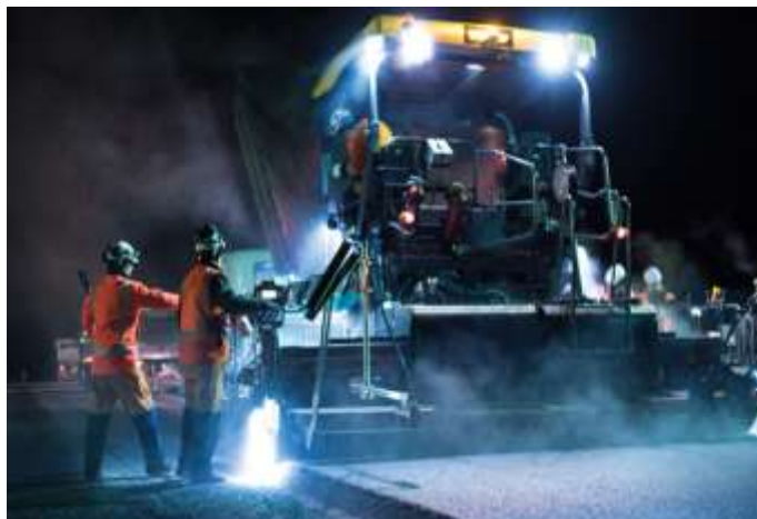
Asphalt overlay work on Lower Queen Street
