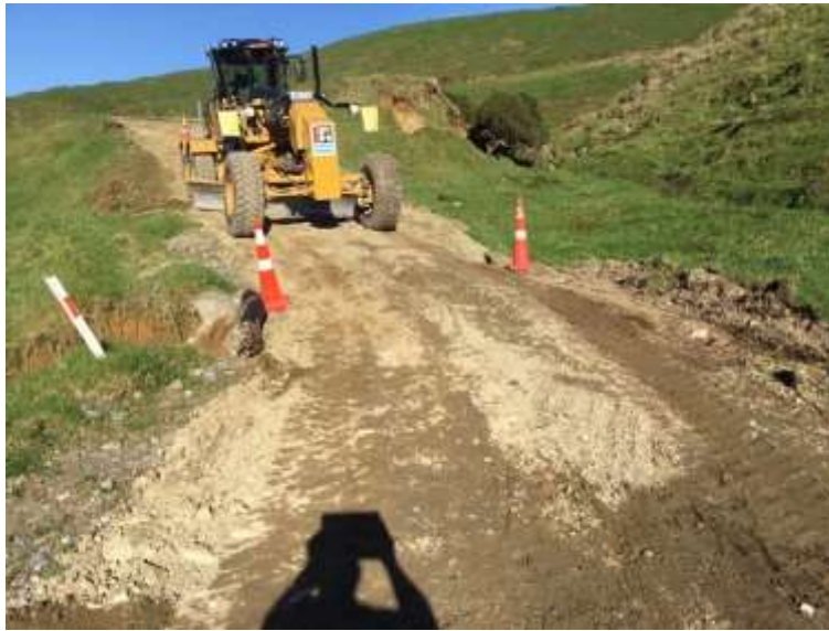
Cowin Road culvert
