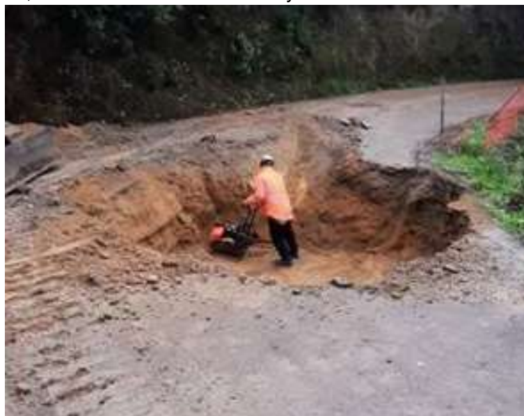
Rosedale Road repair
