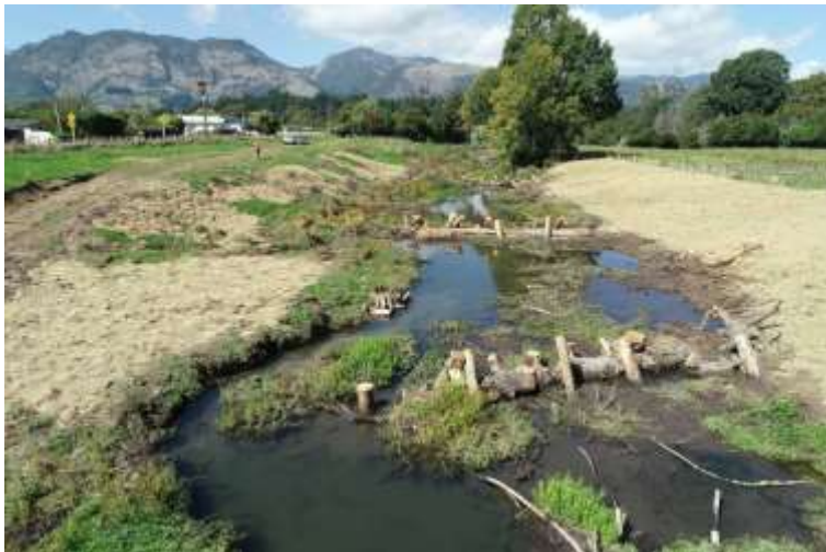
Motupipi River restoration site showing the use of logs for stream management.
