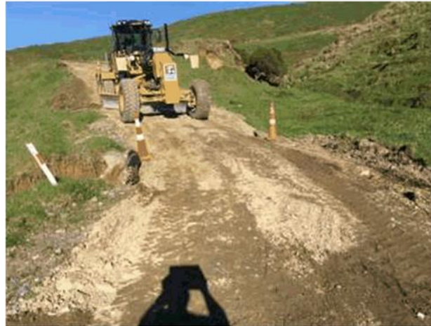
Cowin Road culvert
