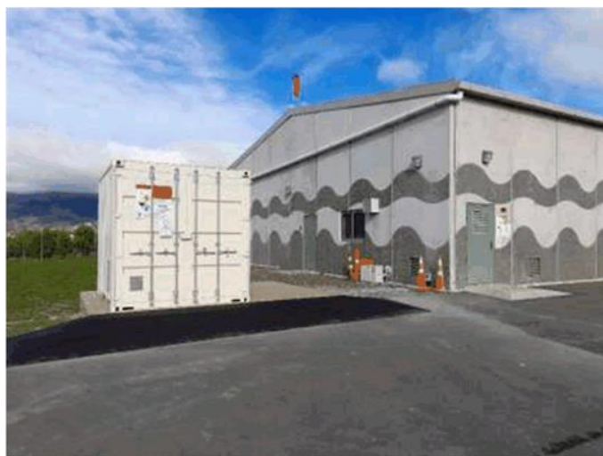
Chlorine storage container, Richmond WTP
