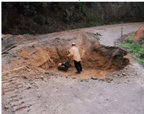
Rosedale Road repair
