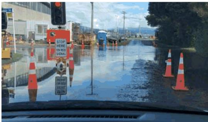
Sea inundation at the corner of Everett Street and Massey Street, Motueka.
