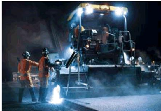
Asphalt overlay work on Lower Queen Street
