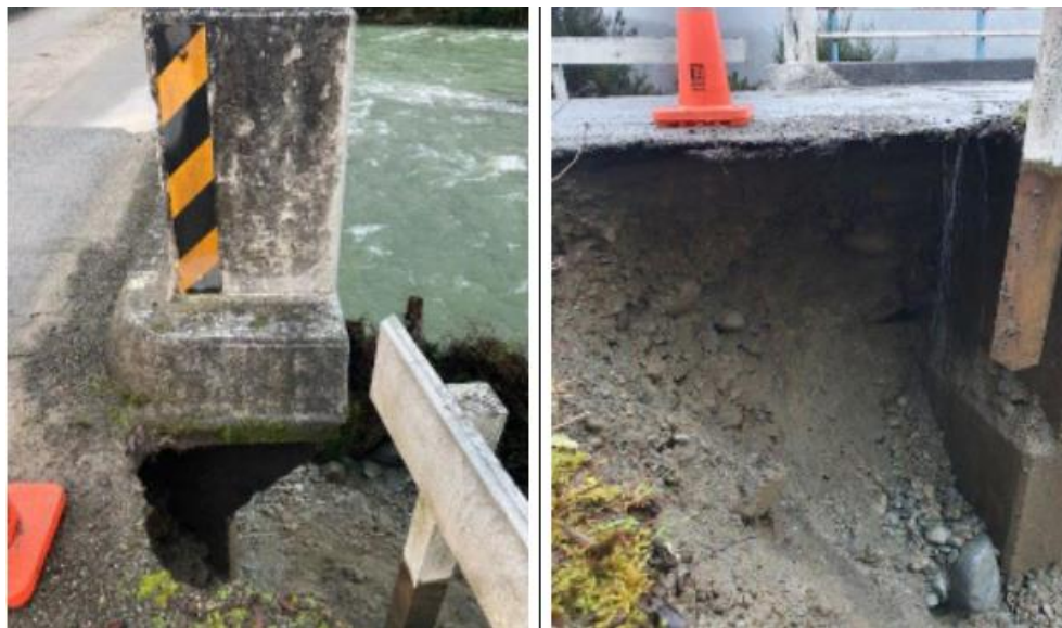
Gowan Valley Road Bridge
