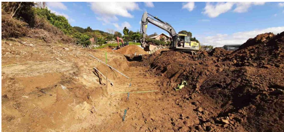
Preparation for installation of stormwater pipes at Pohutukawa Place, Pohara
