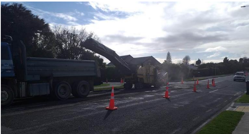
Wensley Road – milling machine in operation
