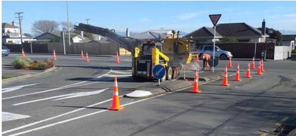
Milling off old surface at William Street intersection
