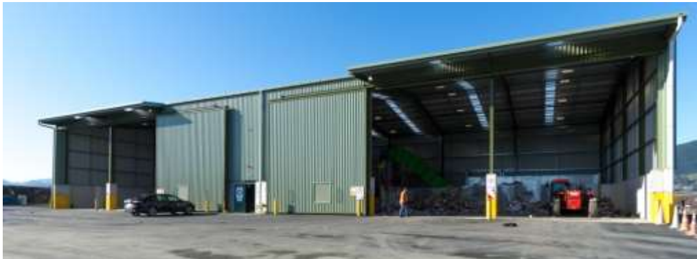
Figure 2: Exterior Photo of Richmond RRC
