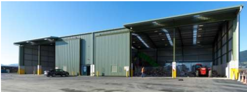
Figure 2: Exterior Photo of Richmond RRC
