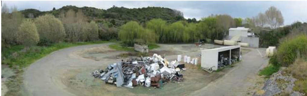
Figure 7: Takaka RRC – from Rear of Site, with Solid Waste Compactor and Bins in Background
