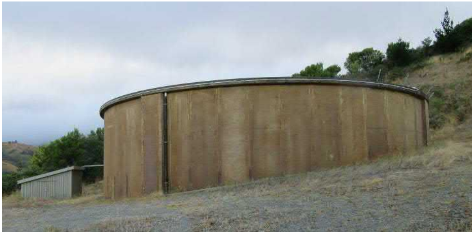
Figure 6-1: Existing water reservoir at Marsden Valley, Stoke, Nelson with 'Permeon' colouration/oxidation process applied to the raw concrete (Photograph taken 3 February 2020, by Noelia O'Leary, design engineer, WSP).
