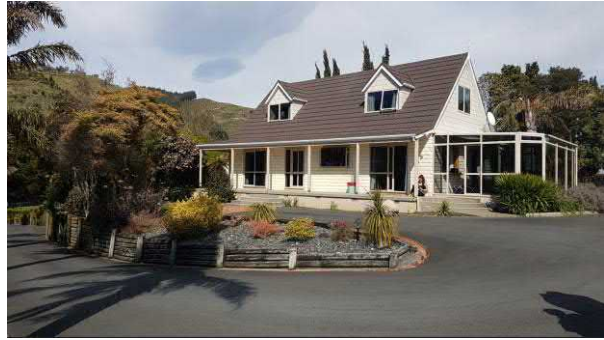
The existing dwelling on site
