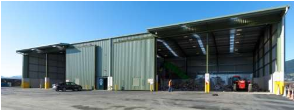
Figure 2: Exterior Photo of Richmond RRC
