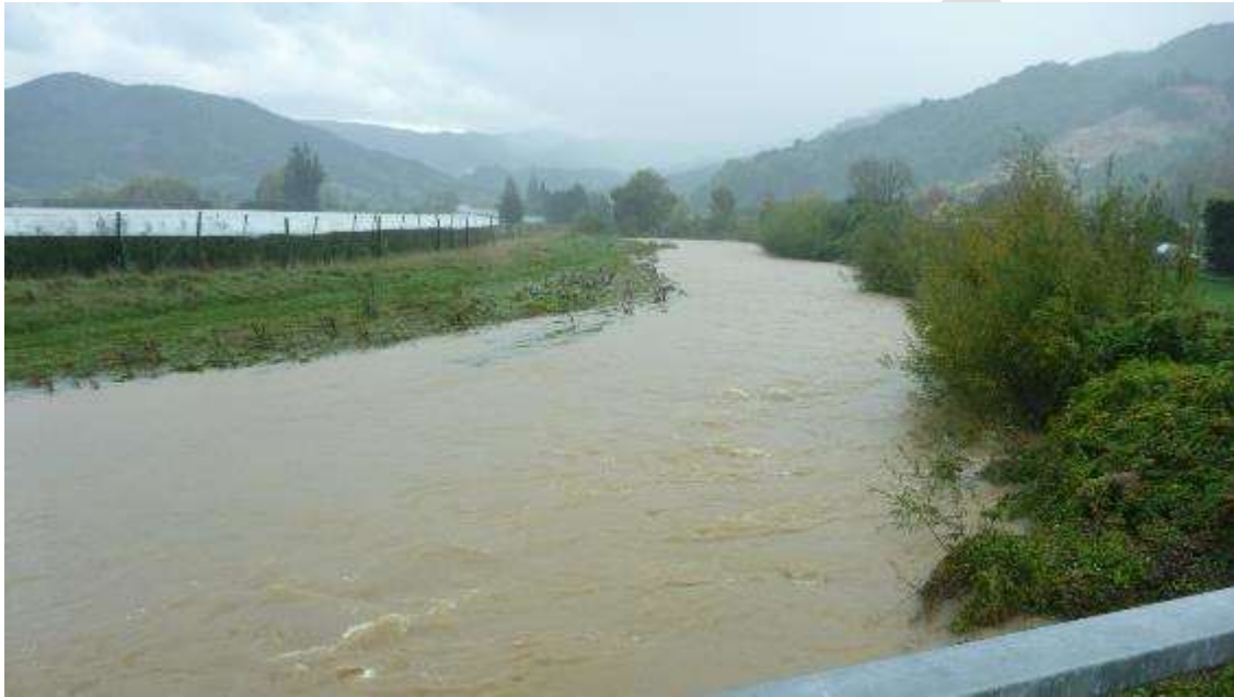
Figure 5: Riwaka River Looking Upstream from the State Highway Bridge
