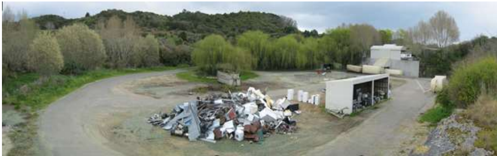
Figure 7: Takaka RRC – from Rear of Site, with Solid Waste Compactor and Bins in Background
