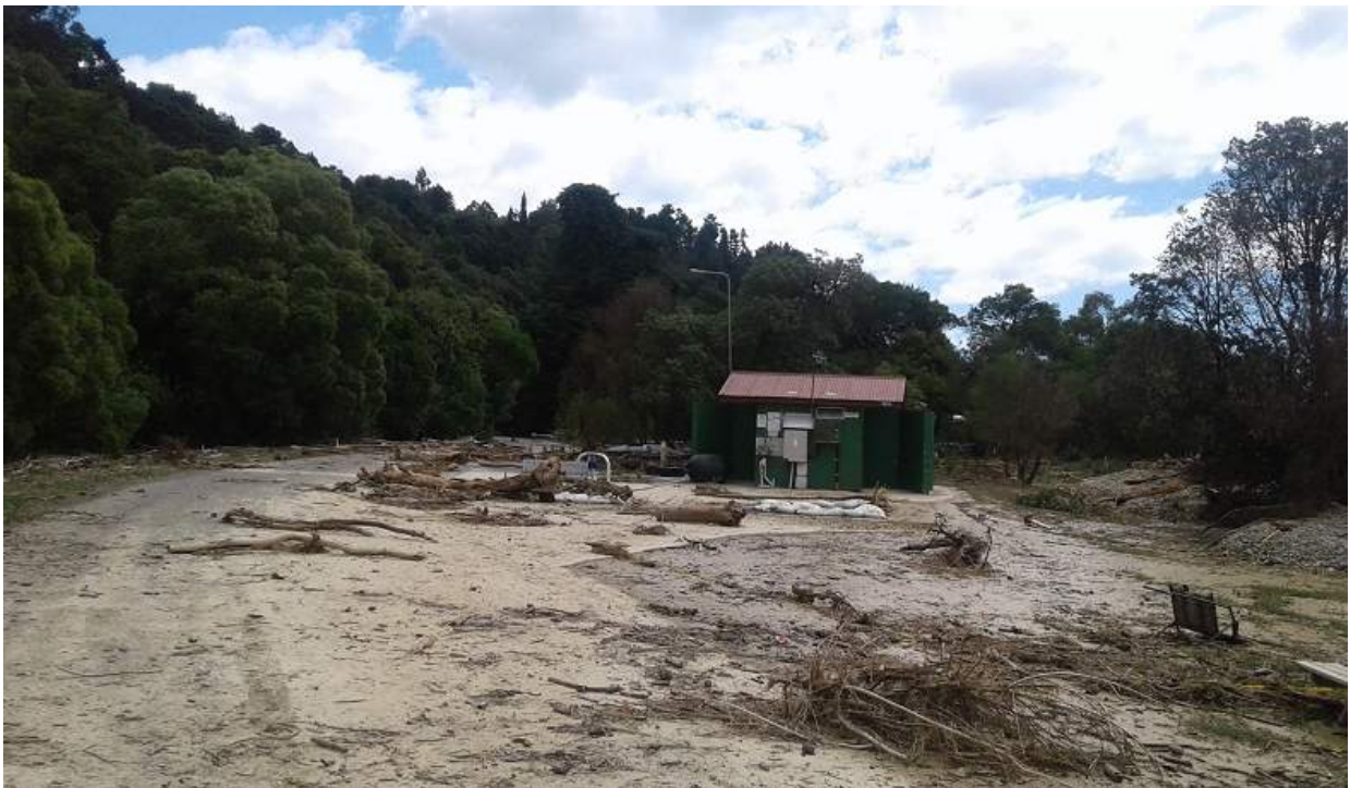
McKee Memorial Recreation Reserve – Toilet Block
