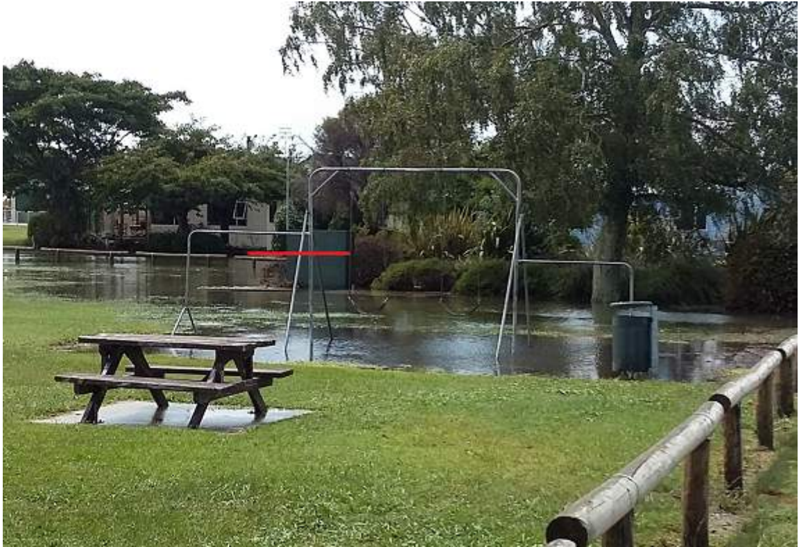
Flooding around Riwaka WWPS (red line marks flood water level)
