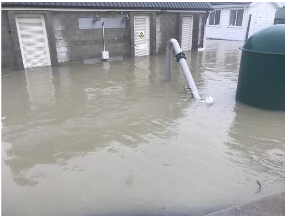
Beach Road WWPS Richmond
