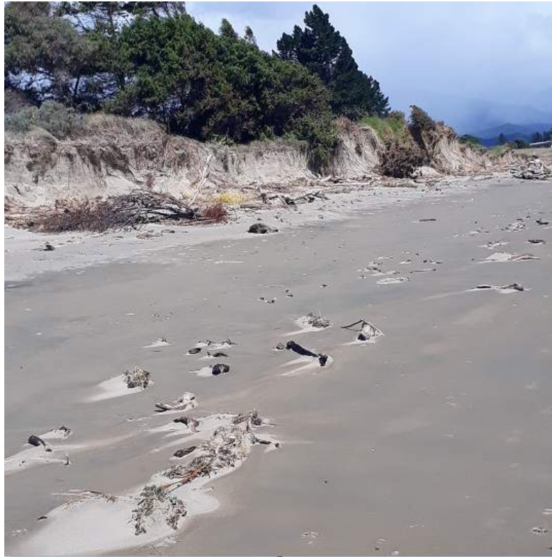
Pohara Beach – Coastal Erosion
