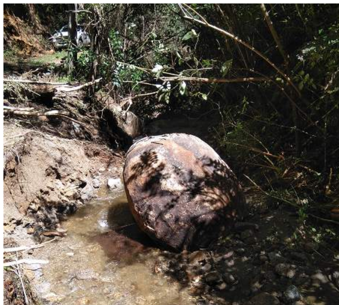
3-4 Tonne Boulder that rolled through intake
