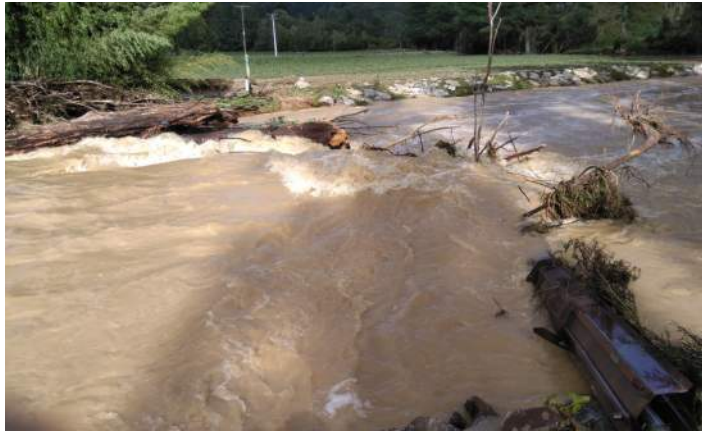
Damaged temporary stream crossing
