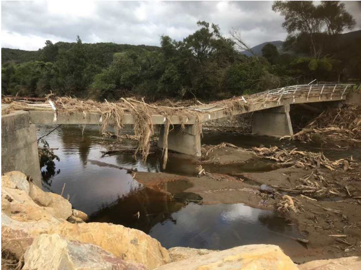
Carter Bridge became a debris trap
