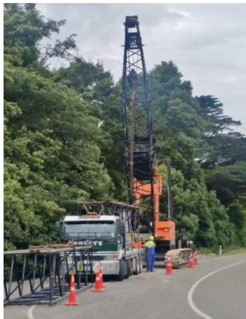
Crane safely delivered to Carter Road to Repair Kaituna Bridge
