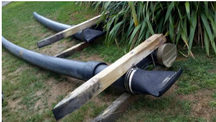
Duckbill Stormwater Outlets – Patons Rock
