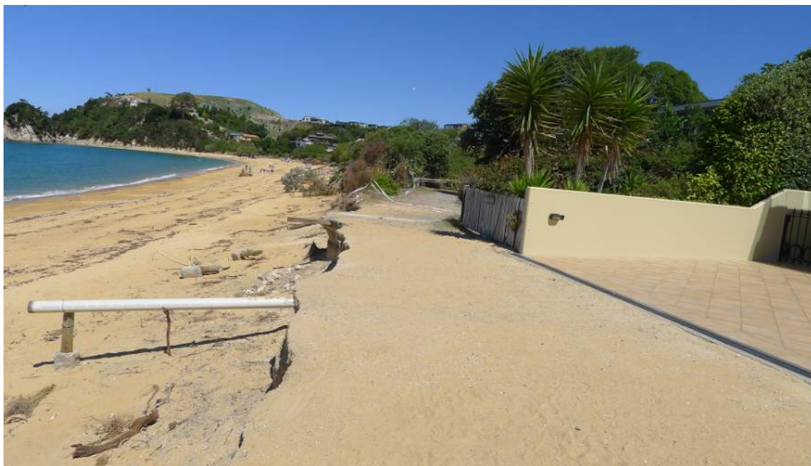
Little Kaiteriteri Beach – Coastal Erosion
