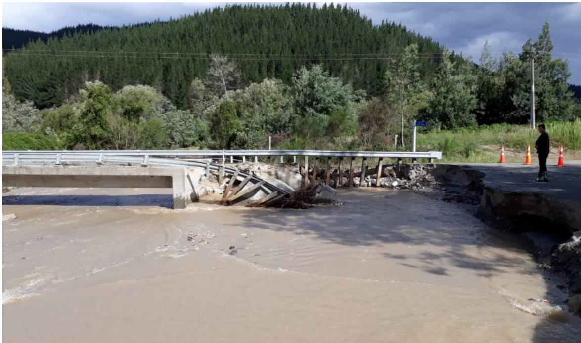
Rocky River Bridge, West Bank Road
