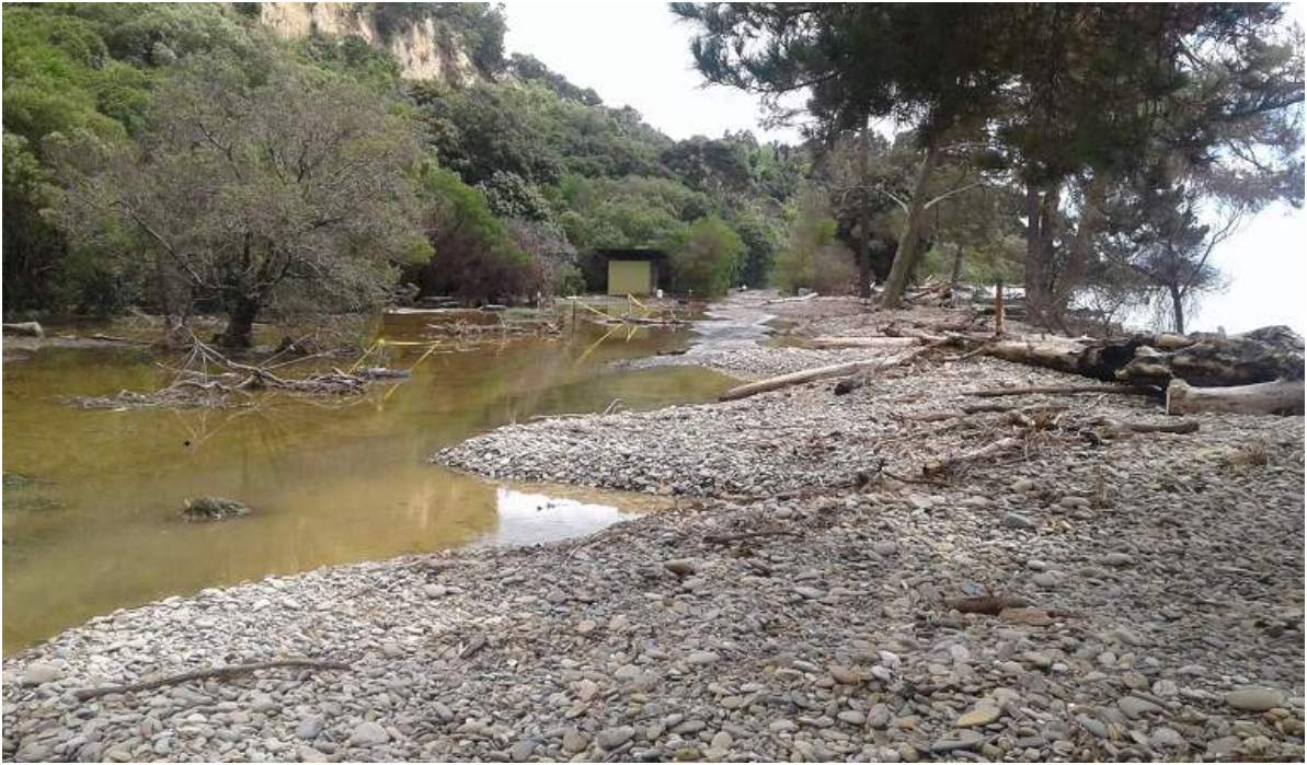
McKee Memorial Recreation Reserve entrance road and toilet block
