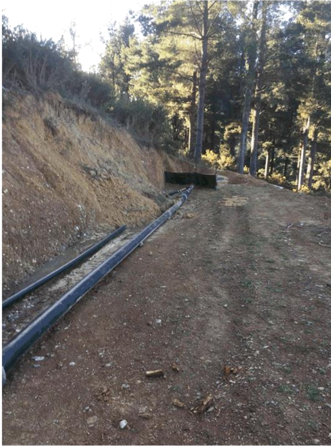
Figure 8.13.4 Side channel of new landfill working area showing sediment fence.
