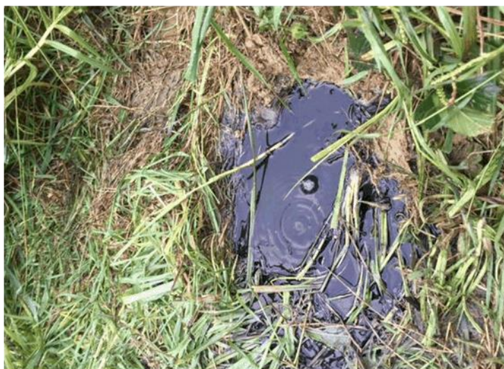
Figure 8.9 Leachate observed during site inspection conducted by Tonkin and Taylor
