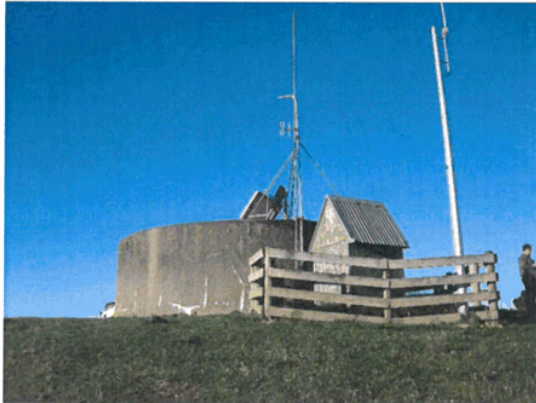
Photo 3-27: View of Silcock’s concrete tank at Dovedale.
