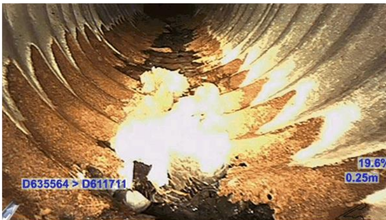
Figure 8.13.4a Condition assessment of storm water main east side of landfill
