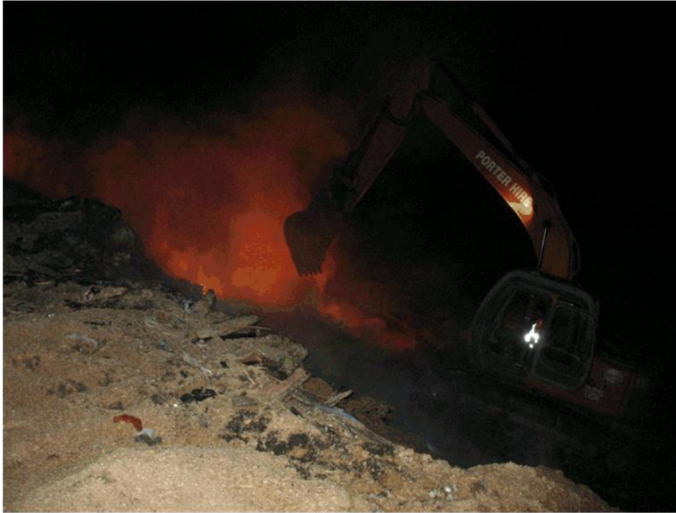
Figure 8.13.9 A fire at the landfill (probably caused by a lithium type battery)
