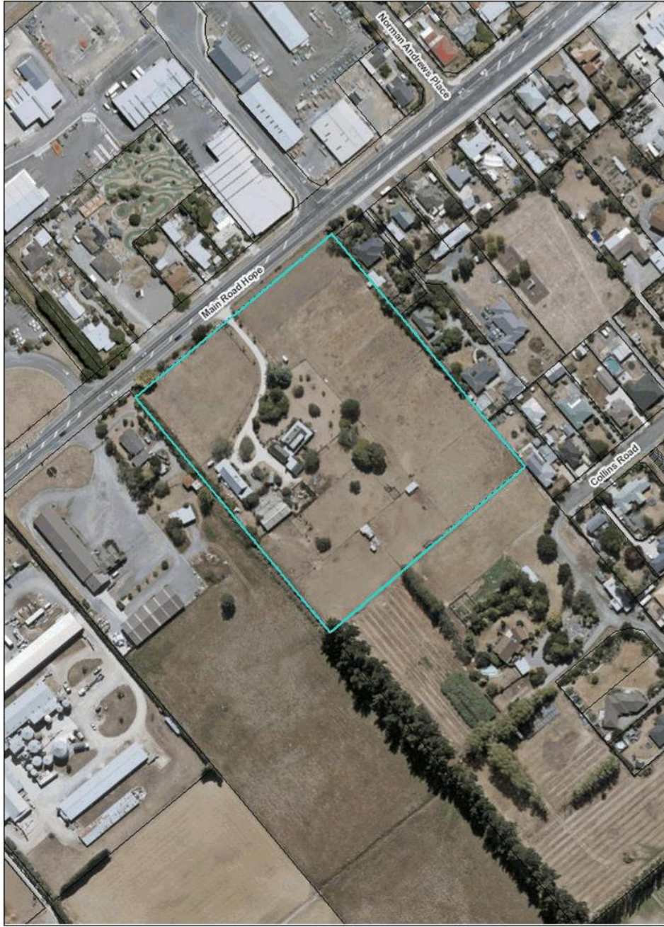
Aerial site photo of the 45 Main Road Hope SHA, Hope
