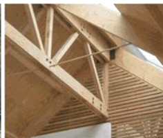
Exposed timber structure
