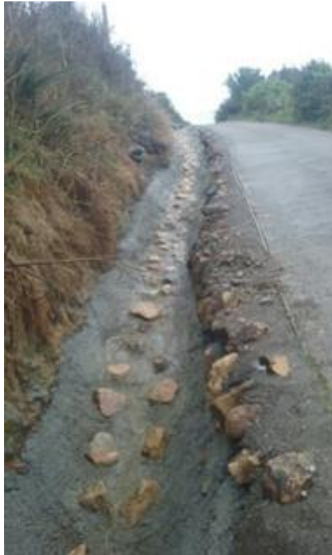
Swiftsure Street concrete and rock lining of channel
