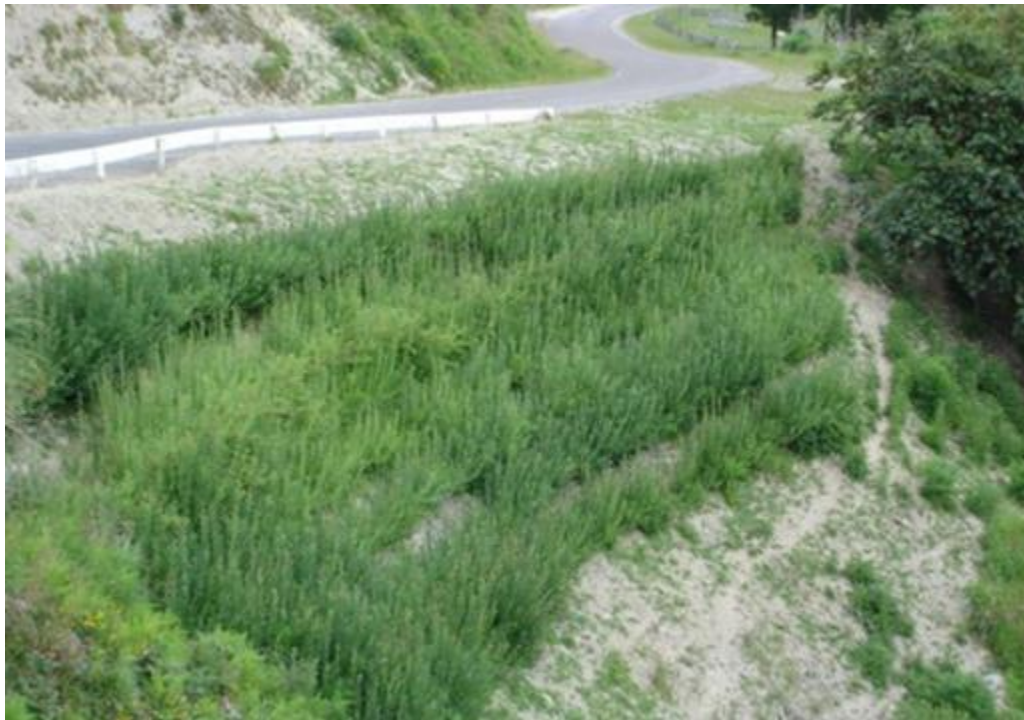
Example of completed walls
