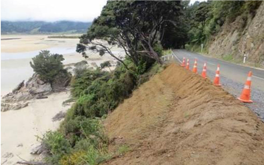
Able Tasman Drive after treatment
