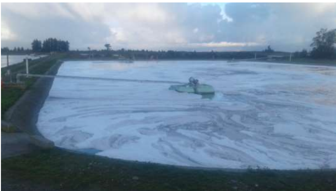
Foaming aeration basin, Motueka - 21 September 2017
