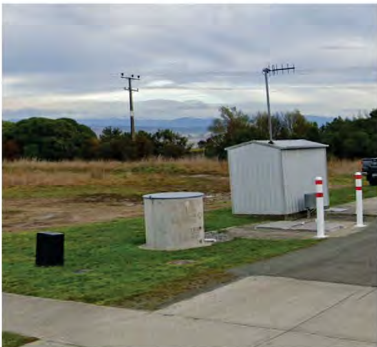
Figure 7-3 Photograph of the Whakatū Pump Station site
