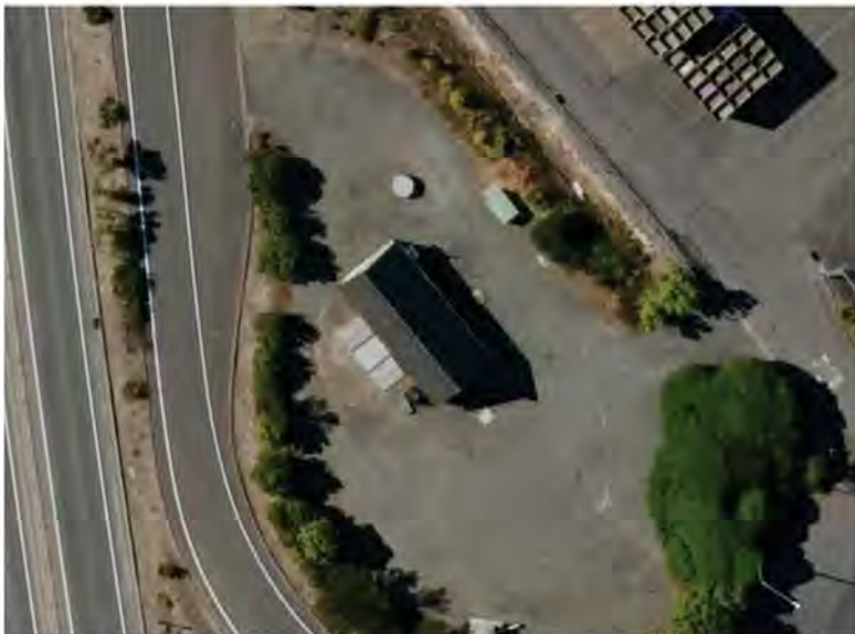
Figure 7-5 Photograph of the Saxton Road Pump Station site
