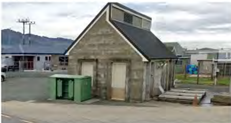
Figure 7-1 Photograph of the Beach Road Pump Station site
