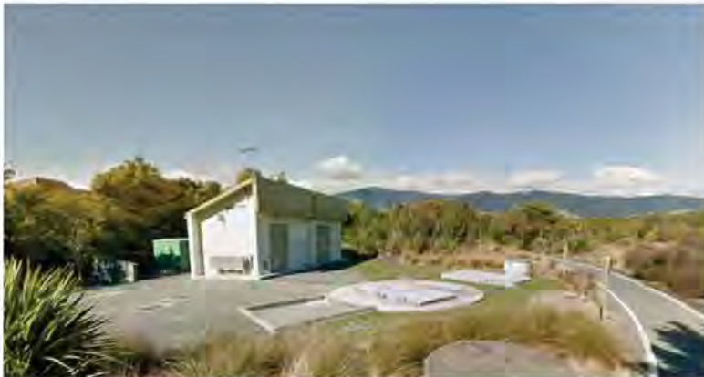
Figure 7-7 Photograph of Songer Street Pump Station site
