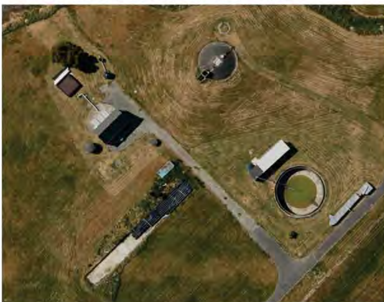
Figure 7-9 Photograph of Airport Pump Station site
