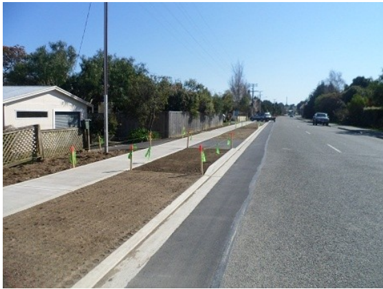
Aranui Road upgrade
