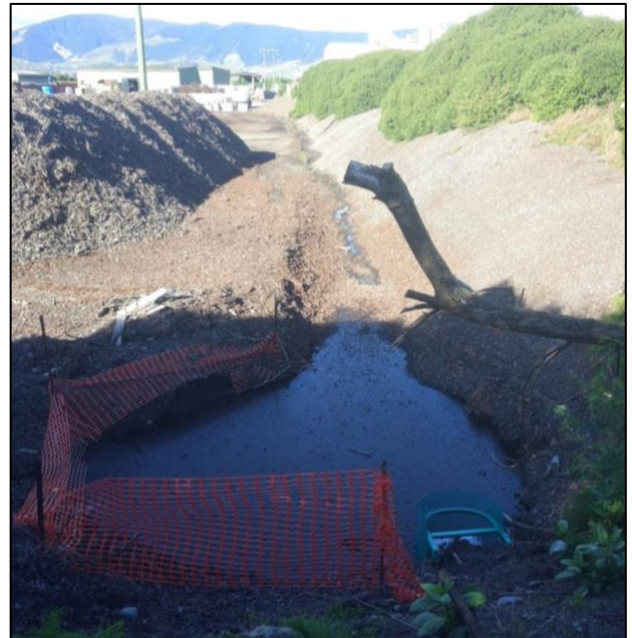
Site water discharges from the south-western side of the Bark Processor's facility directly to the estuary via a piped outlet.
