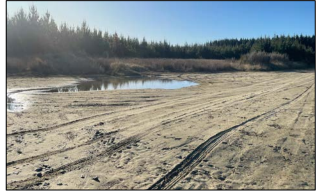
Roadway blocking site from regular tidal inundation. Note fresh deposits of sand from spring tide inundation.
