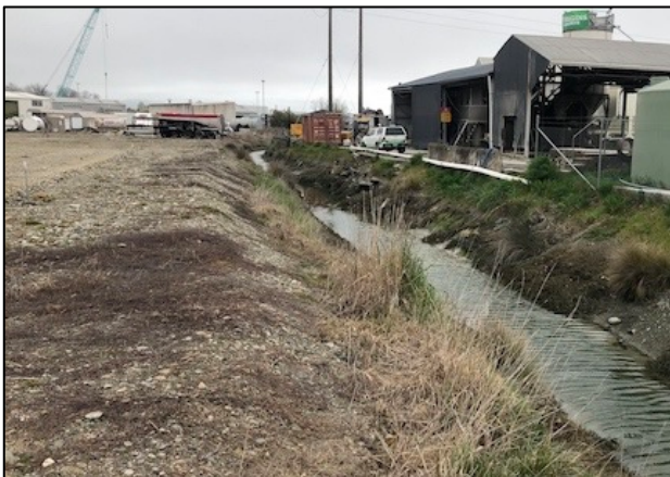
Vercoes Drain showing channelisation and surrounding landuse. Note the presence of salt marsh along the channel edge.
