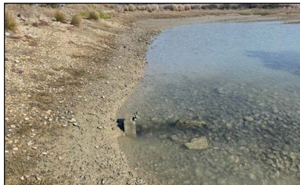
Small pipe and flap gate restricting tidal flows to the site.
