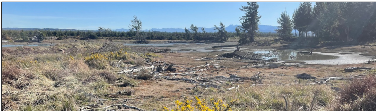
Tidal water and pine slash trapped behind the historical causeway. The grassy area to the left of the picture has recently been cleared of mature pine trees.
