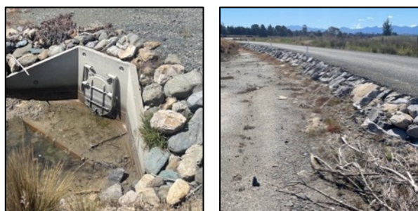
Flap-gate and causeway limiting tidal exchange to the site.
