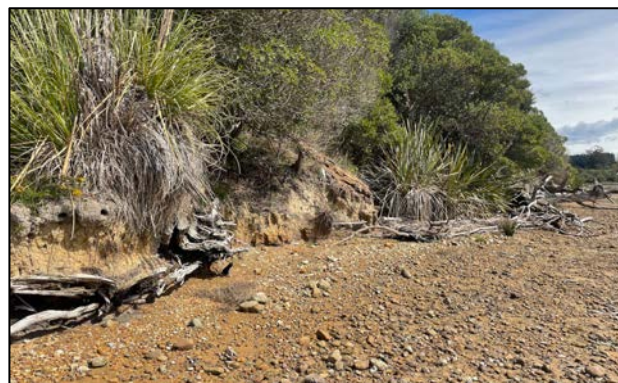
Eroding terrestrial edge of the site.
