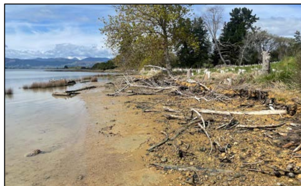
Eroding clay margin with debris from recent pine felling.
