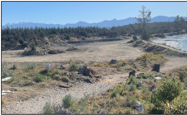
Coastal berm and walkway/cycleway with new (early 2023) raised berm to prevent tidal inundation on the seaward edge.
