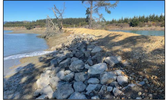
Riprap reinforced culvert and berm at culvert discharge point.
