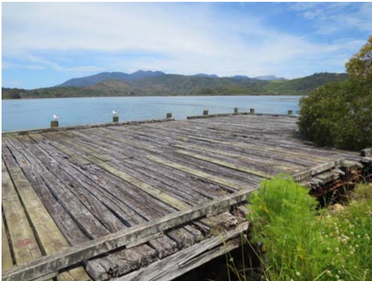
Photograph 22: Existing Milnthorpe Quay structure.
