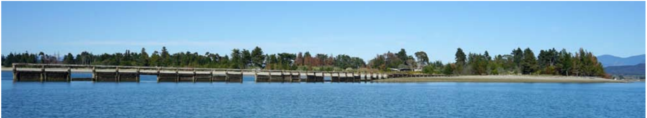
Photograph 73: Northern end of Jackett Island (groyne visible in foreground). Port Motueka to the right (outside of field of view).
