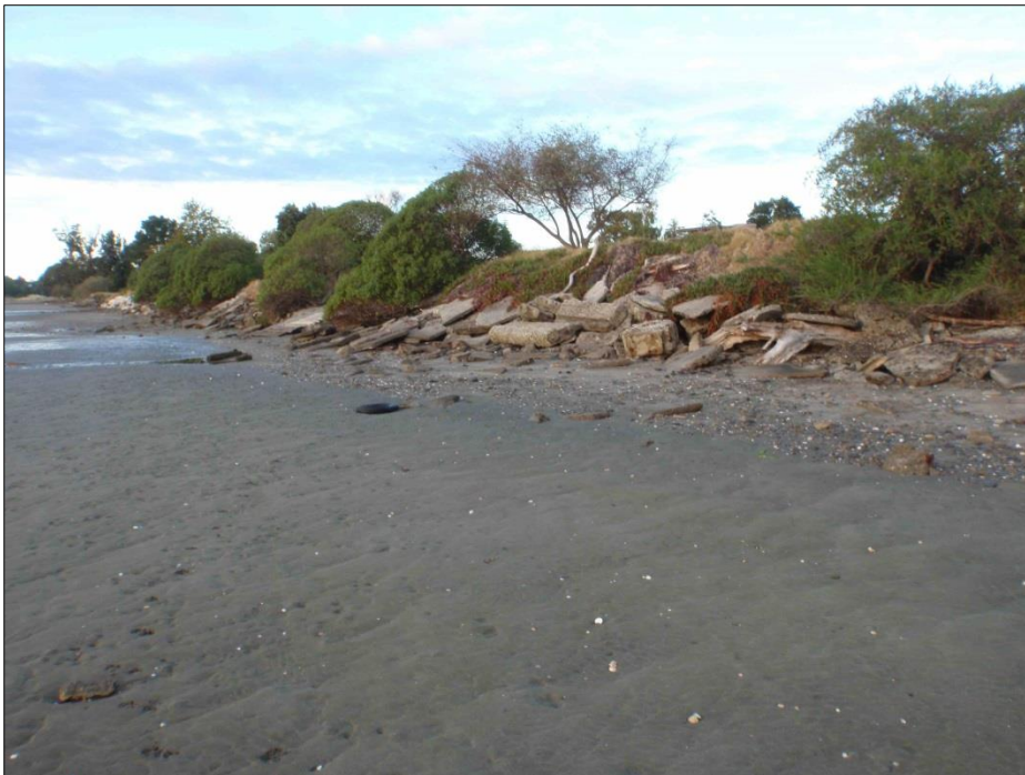
Plate 5. Moutere delta erosion protection.
