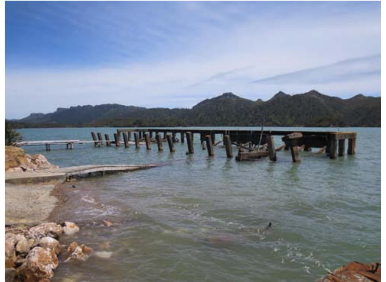
Photograph 14: Typical character of existing wharf.
