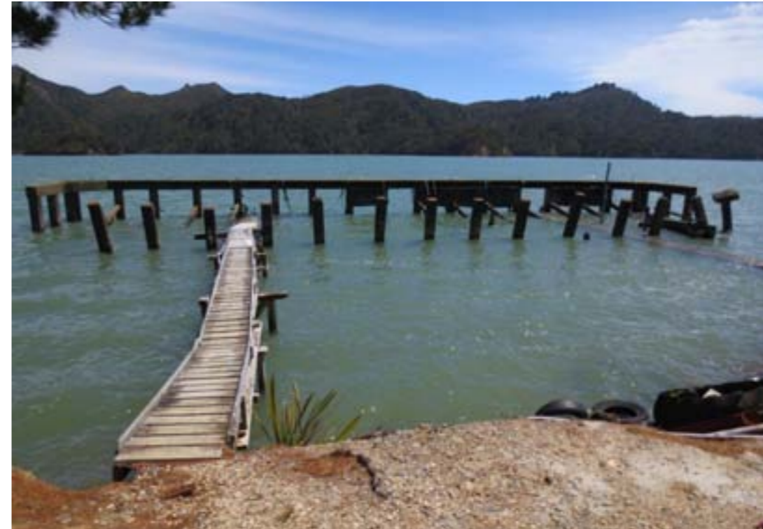
Photograph 10: Typical character of existing wharf.
