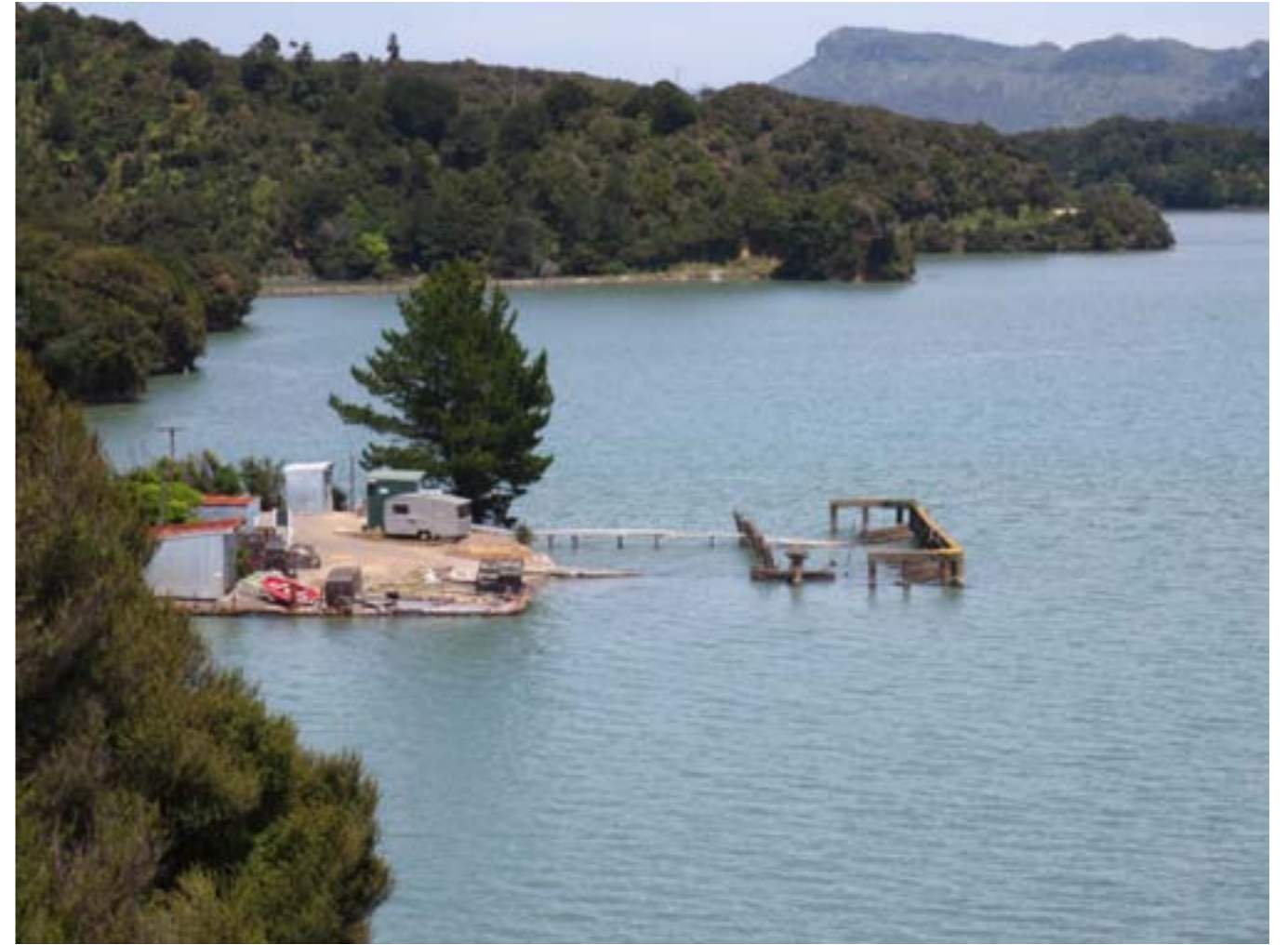
Photograph 16: Zoomed in view out over wharf.
