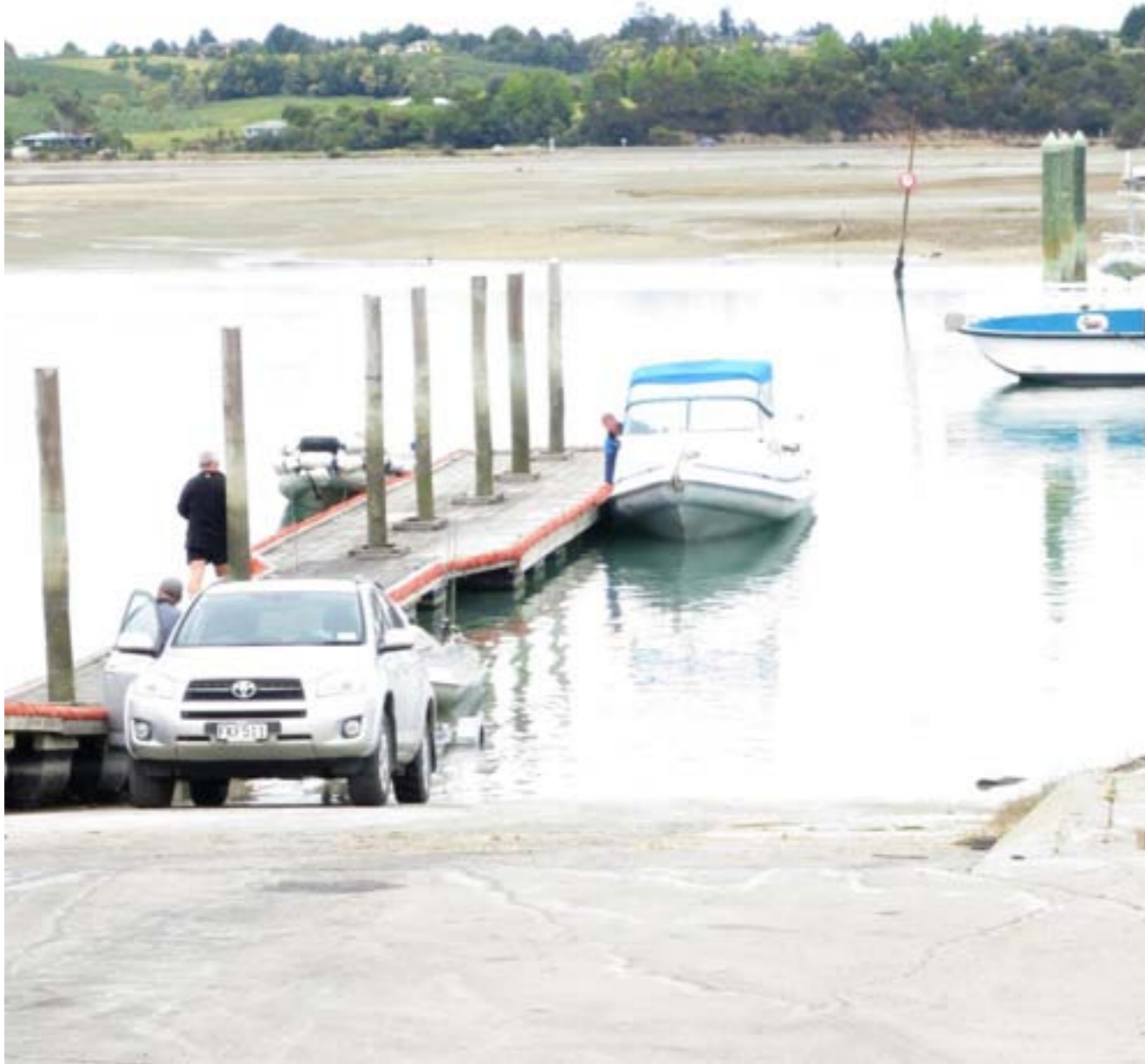
Photograph 80: Typical character of proposed mooring area as seen from the marina.
