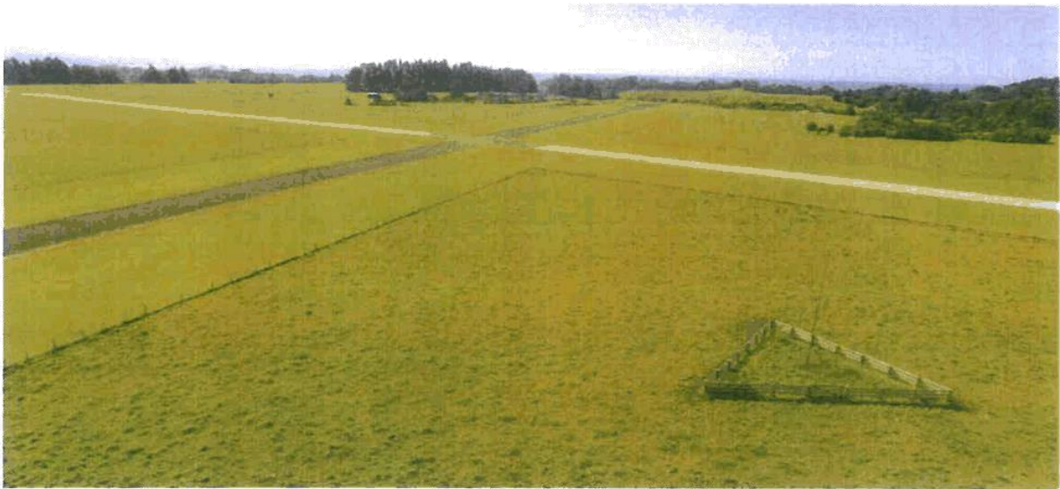
WEATHER STATION AND VIEW OF 11/29 THAT NEEDS SEAL
