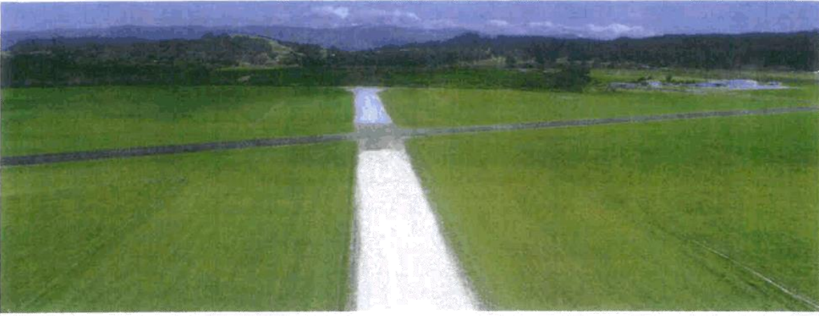
RUNWAY 11/29 THAT REQUIRES SEALING
