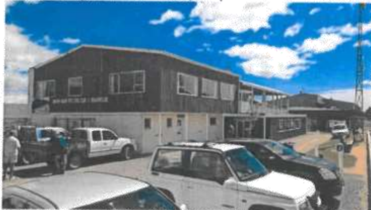
Figure 2 - View from the South West, 2017
