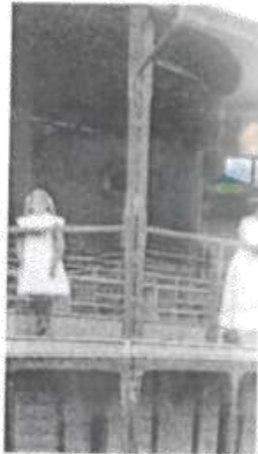
Figure 19 - Close up of Post from c1911 image, source GBSGSC
