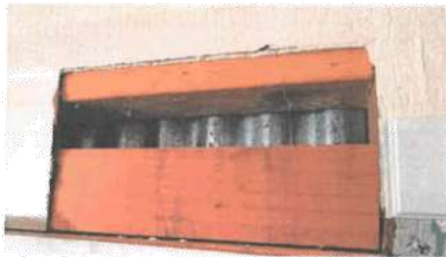
Figure 5 - Corrugated Iron exterior cladding at old opening west doorway
