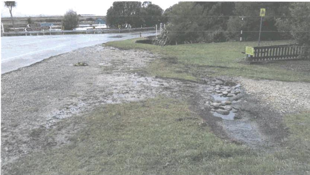
Takaka-Collingwood Highway at Collingwood: Junction of SH60 with local roads at "Zatori" corner, showing walkway exit area which is shared between pedestrians, carparking and stormwater.
