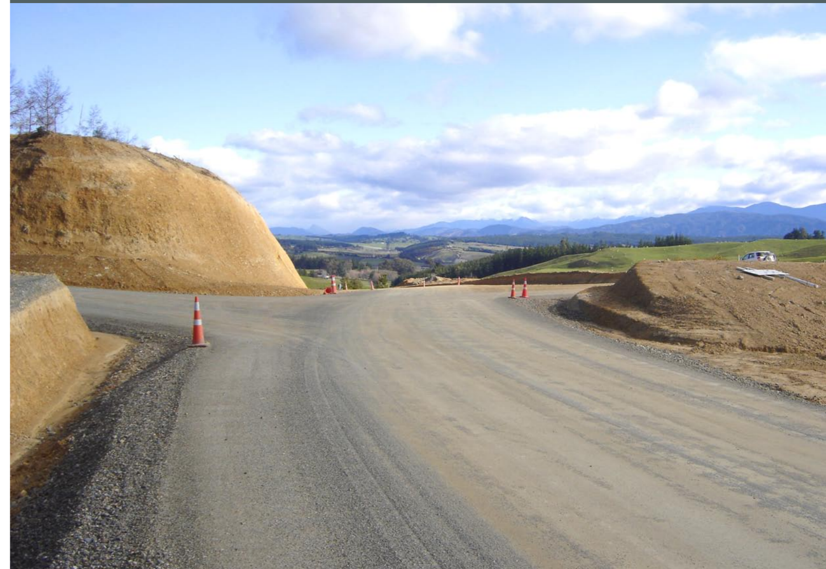
Intersection of Harley Road and Old Coach Road.
