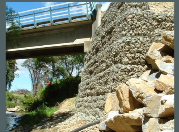
Sherry Road Bridge.
