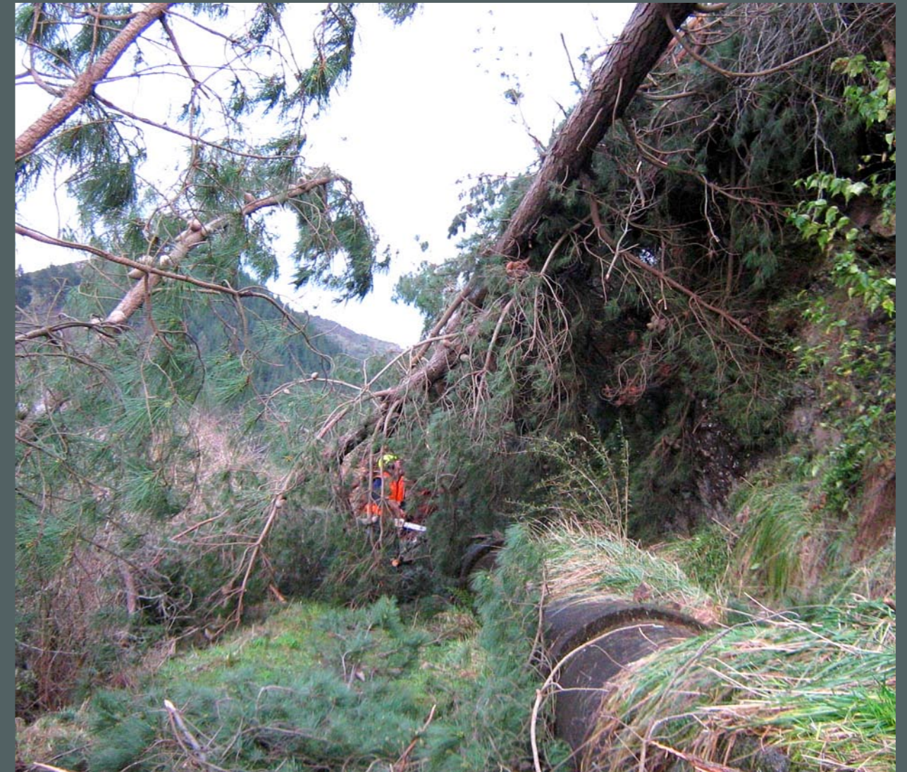
Repairing the Maitai pipeline.
