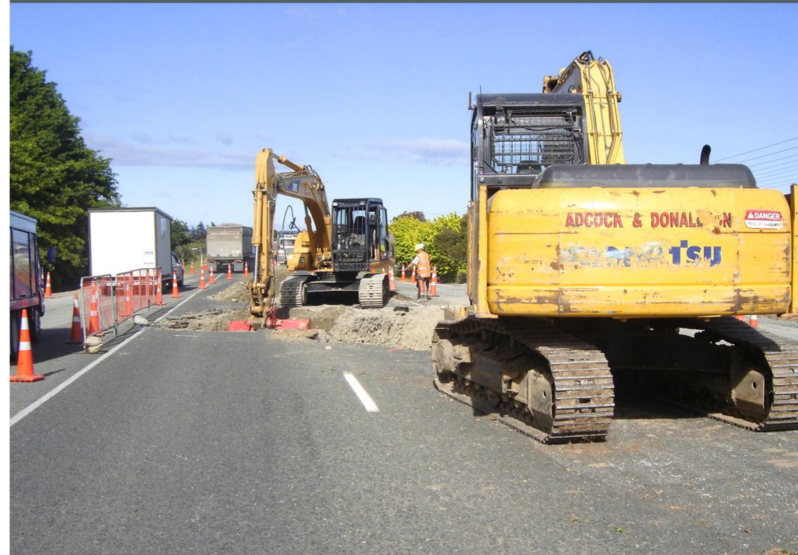
Laying stormwater pipe at Richmond Deviation.
