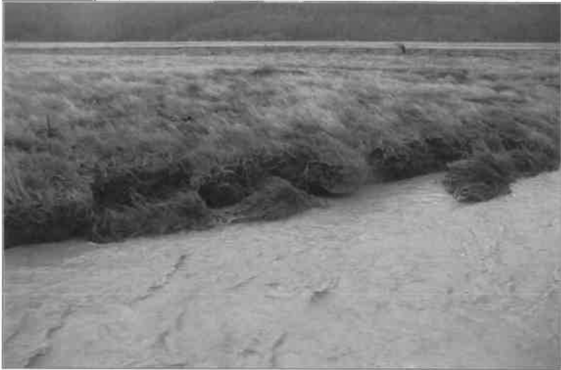
Figure 23 Site 3 bank failure at 95 m 3 /s (2013 May 26)
