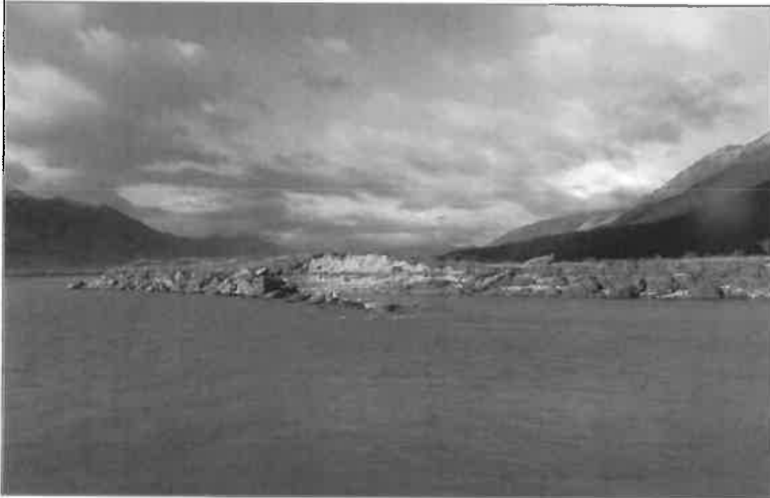
Figure 17 Site 5 eroded stopbank (2013 May 25)
