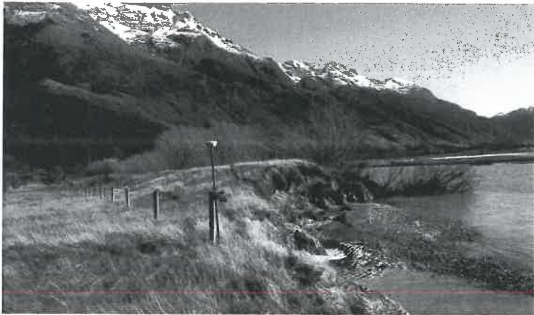
Figure 37 Erosion of the eastern end of the stopbank at site 6 (6 June 2013)
