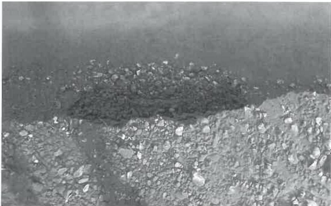
Figure 19 Site 4 irregular local gravel bar scarp collapse
