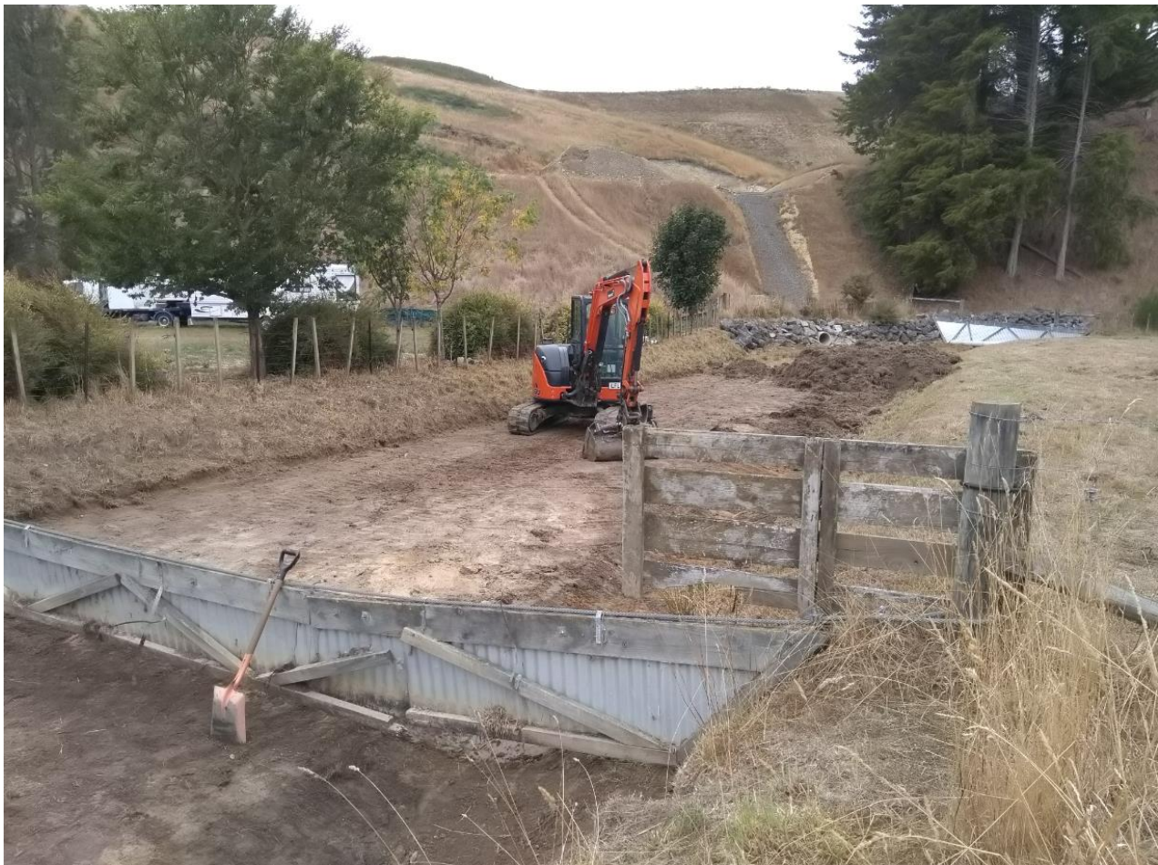
Removal of silt from Jeffries Creek, Lord Rutherford Road South, Brightwater
