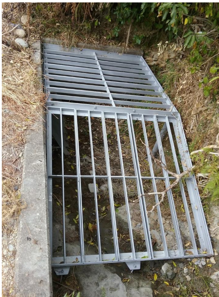
Culvert inlet grill – Gibbs Road, Collingwood
